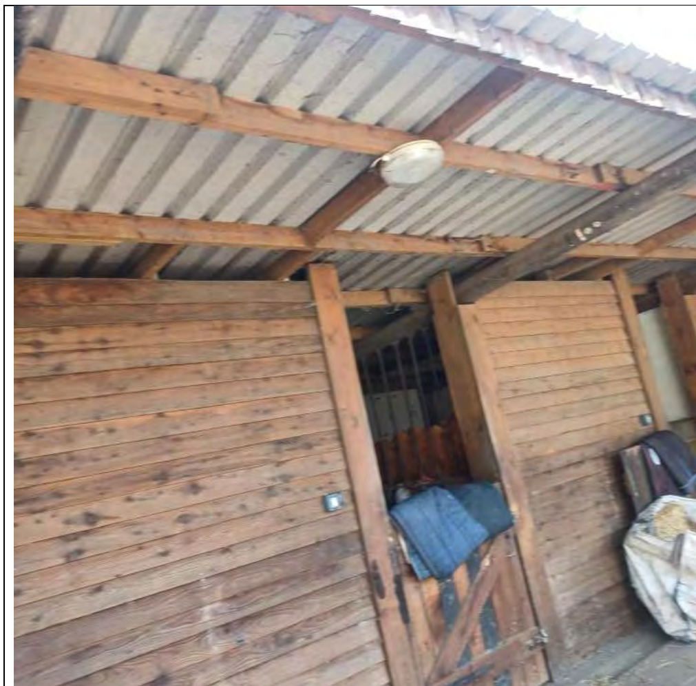
Plate 26: Suspected asbestos cementitious sheeting above fence
