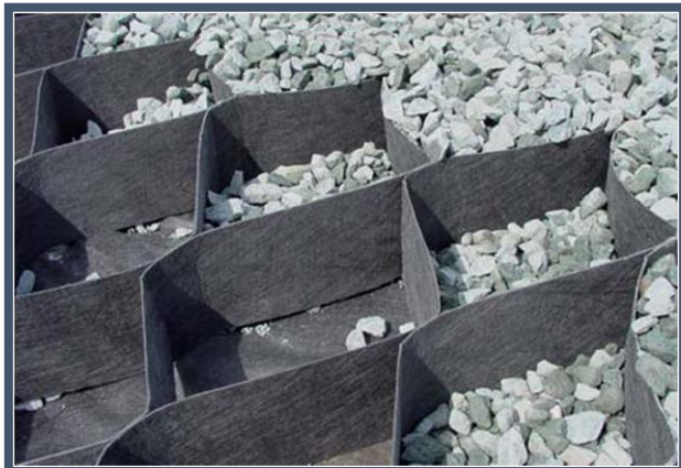
Figure 10 Examples of Cellweb filling with angular stone
