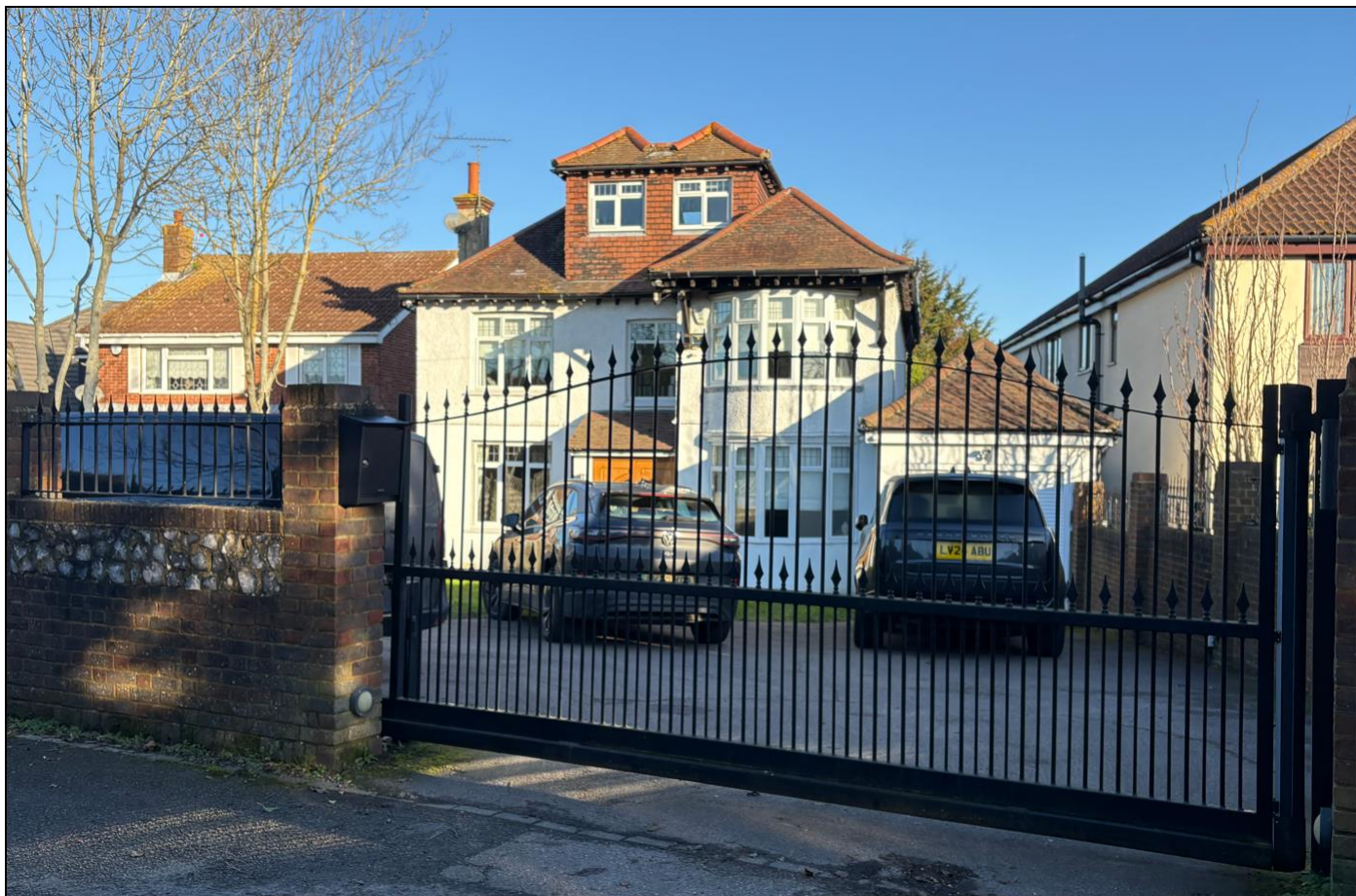
Site Visit Photograph
