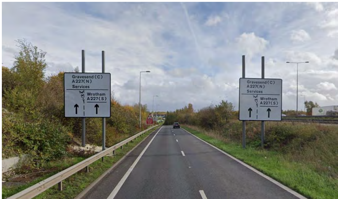
Figure 4.2 Advanced Signage – A2 Eastbound Off Slip
