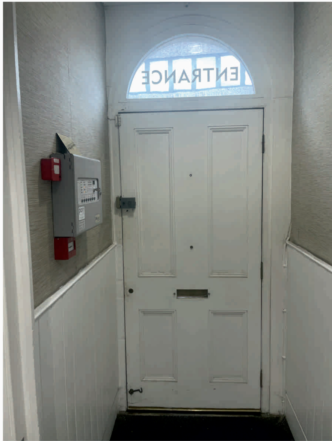
PORCH LOBBY 4 - Looking toward original entrance door curved fanlight and wainscoting all to remain. Note fire alarm control panel
