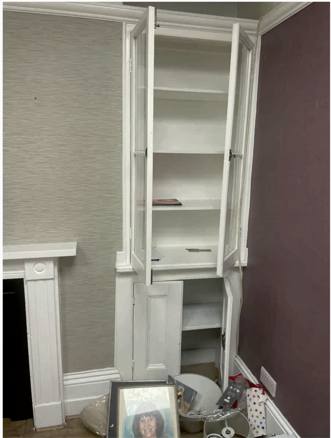
ROOM 6 - Right hand original built in cupboard and display cabinet with original picture rail and skirting
