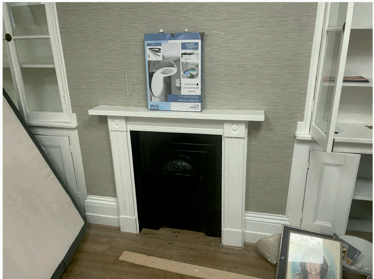
ROOM 6 - Central original fire place and surround to remain intact with original skirting
