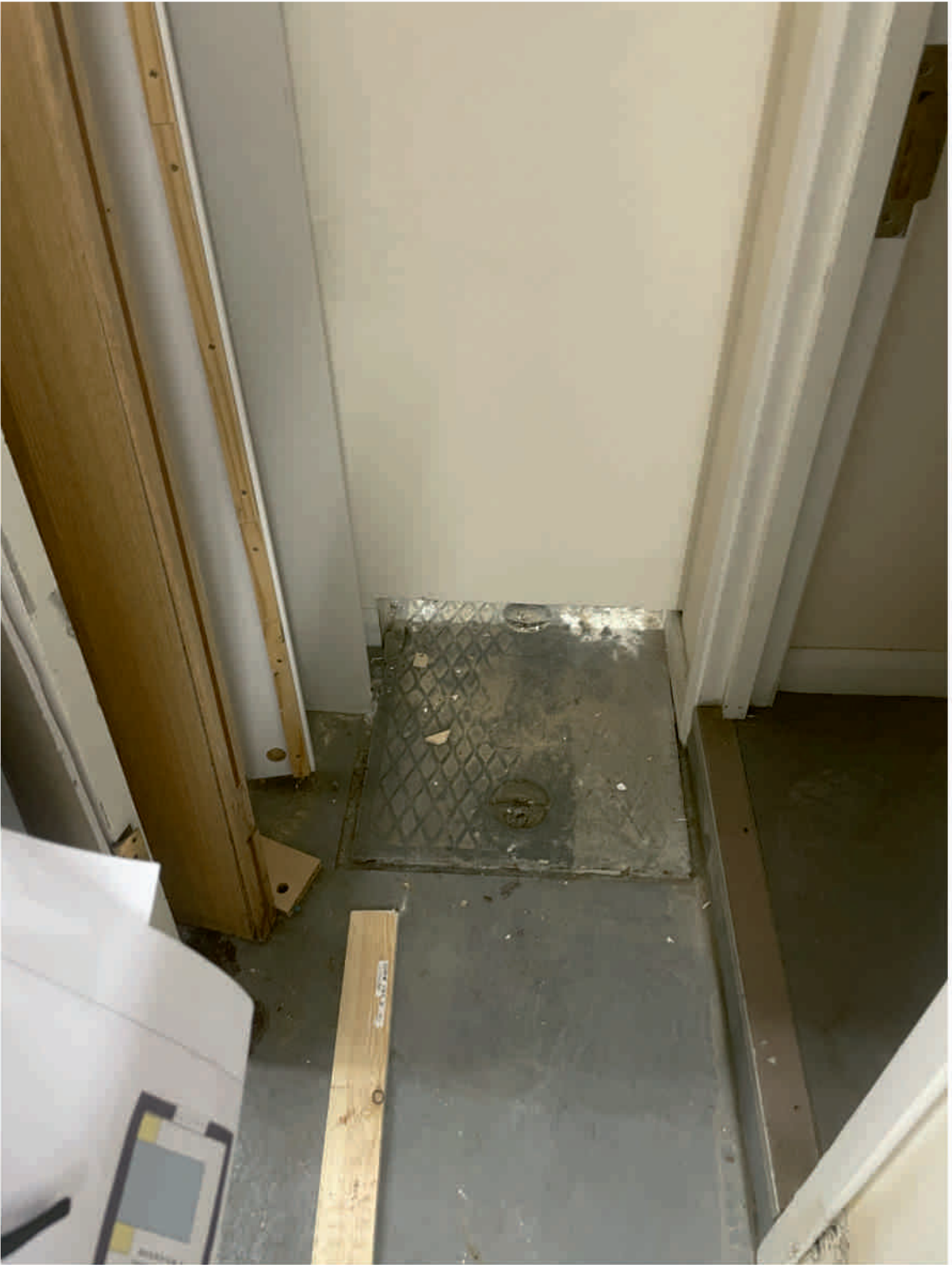
ROOM 9 - Showing internal inspection chamber under new partition!
