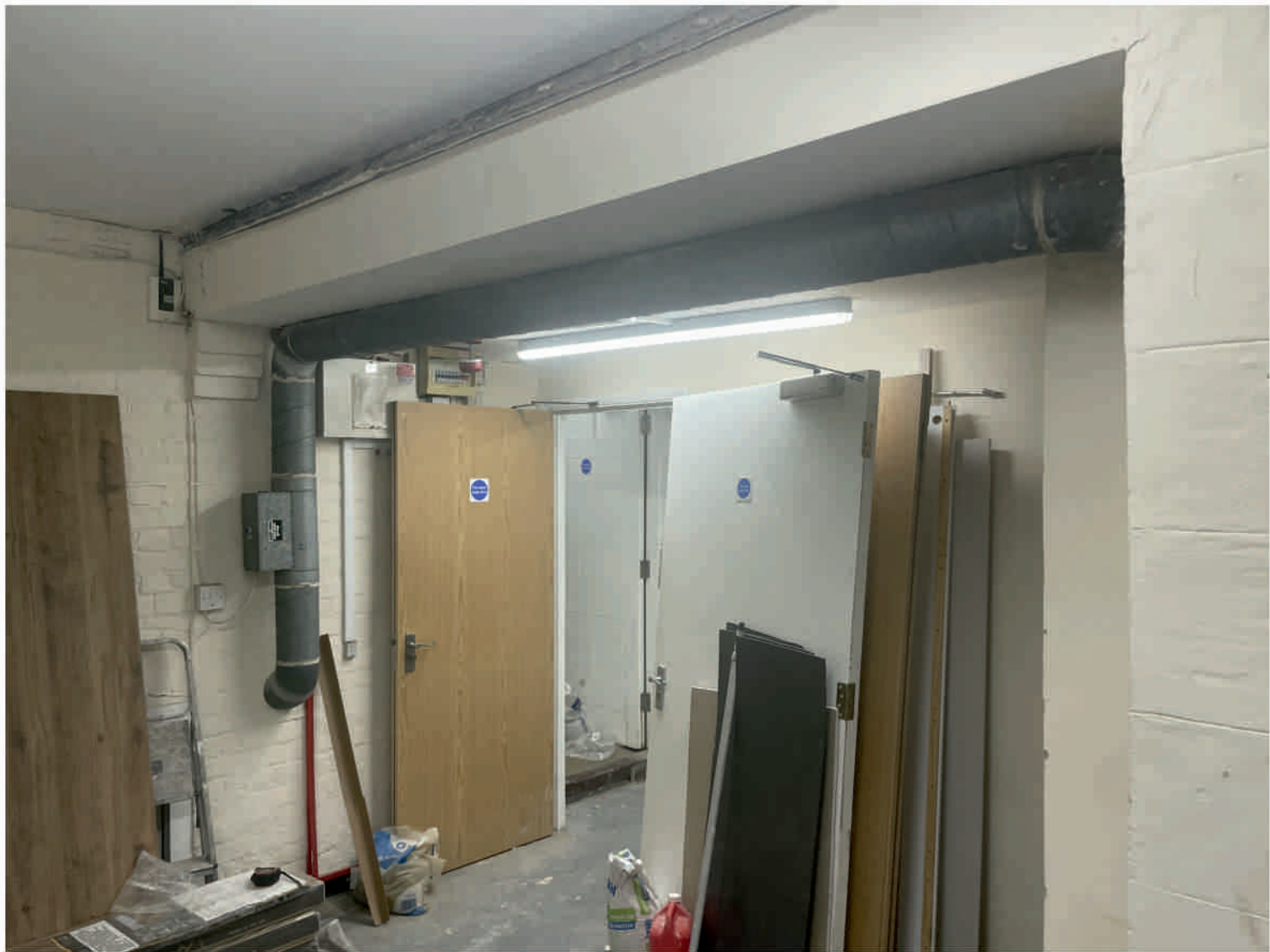
ROOM 9 - Looking back from room 9 toward entrance from room 7. No original features.
