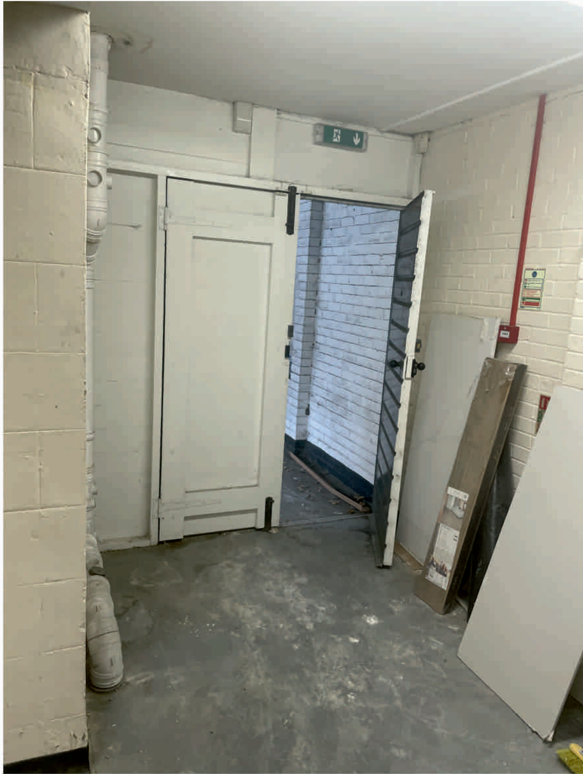
ROOM 9 - Looking toward rear doors to exterior no original features
