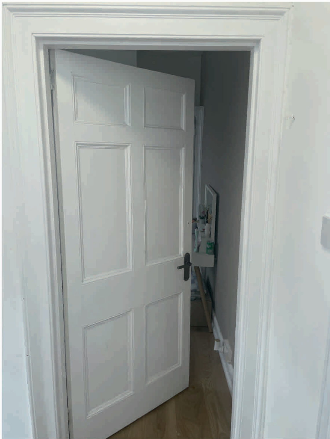
STAIR ENCLOSURE 15 - Looking at entrance door to room 19 from first floor landing. Original door and architrave to be retained but will need to be 30min FR
