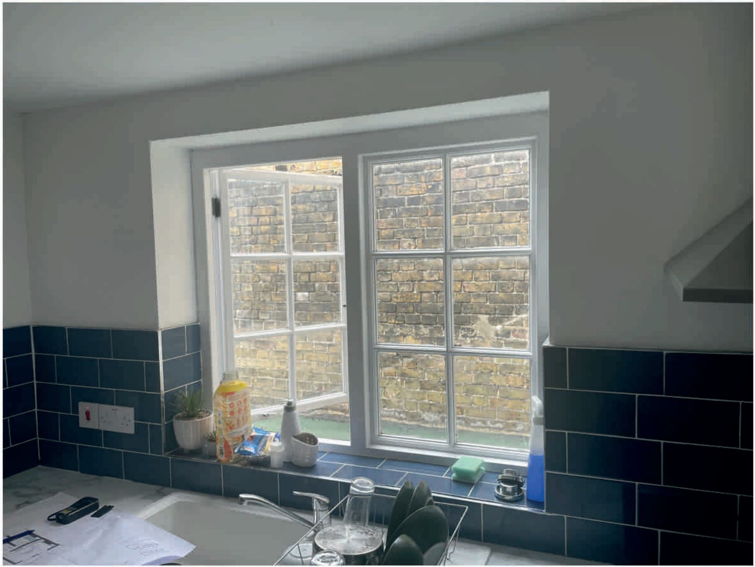
ROOM 16 - Showing non original but matching window.
