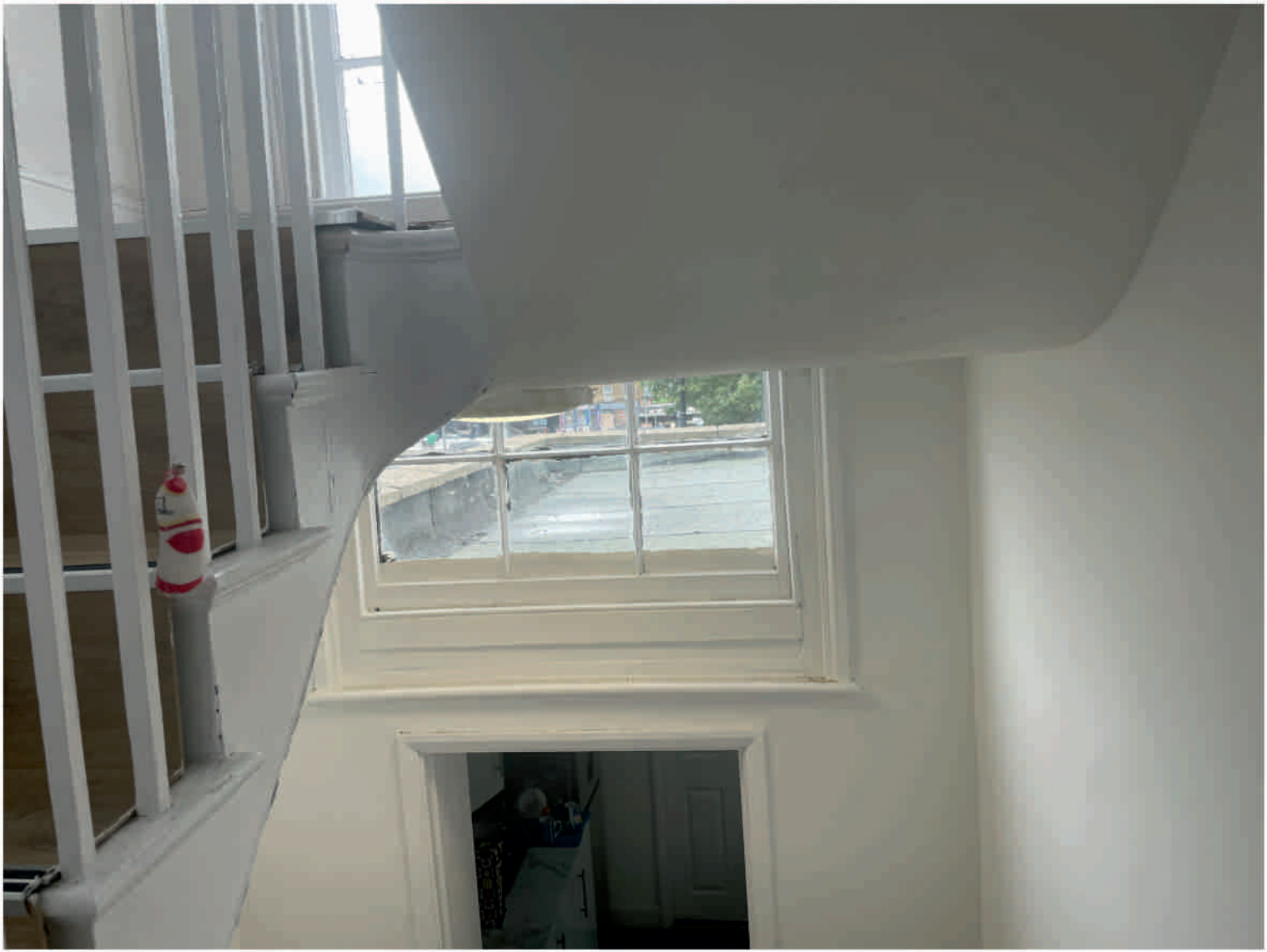
STAIR ENCLOSURE 15 - From fist floor landing to original rear top hung window below second floor flight below half landing. Door to room 16 is shown also. Original final flight of stair can be seen with cut string, nosing and balusters all to remain.
