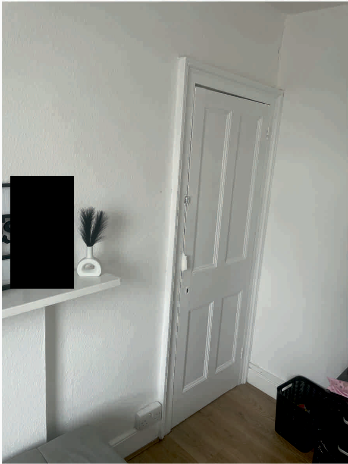
ROOM 21 - Original built in cupboard right hand corner. Note, no fireplace but the mantel remains.
