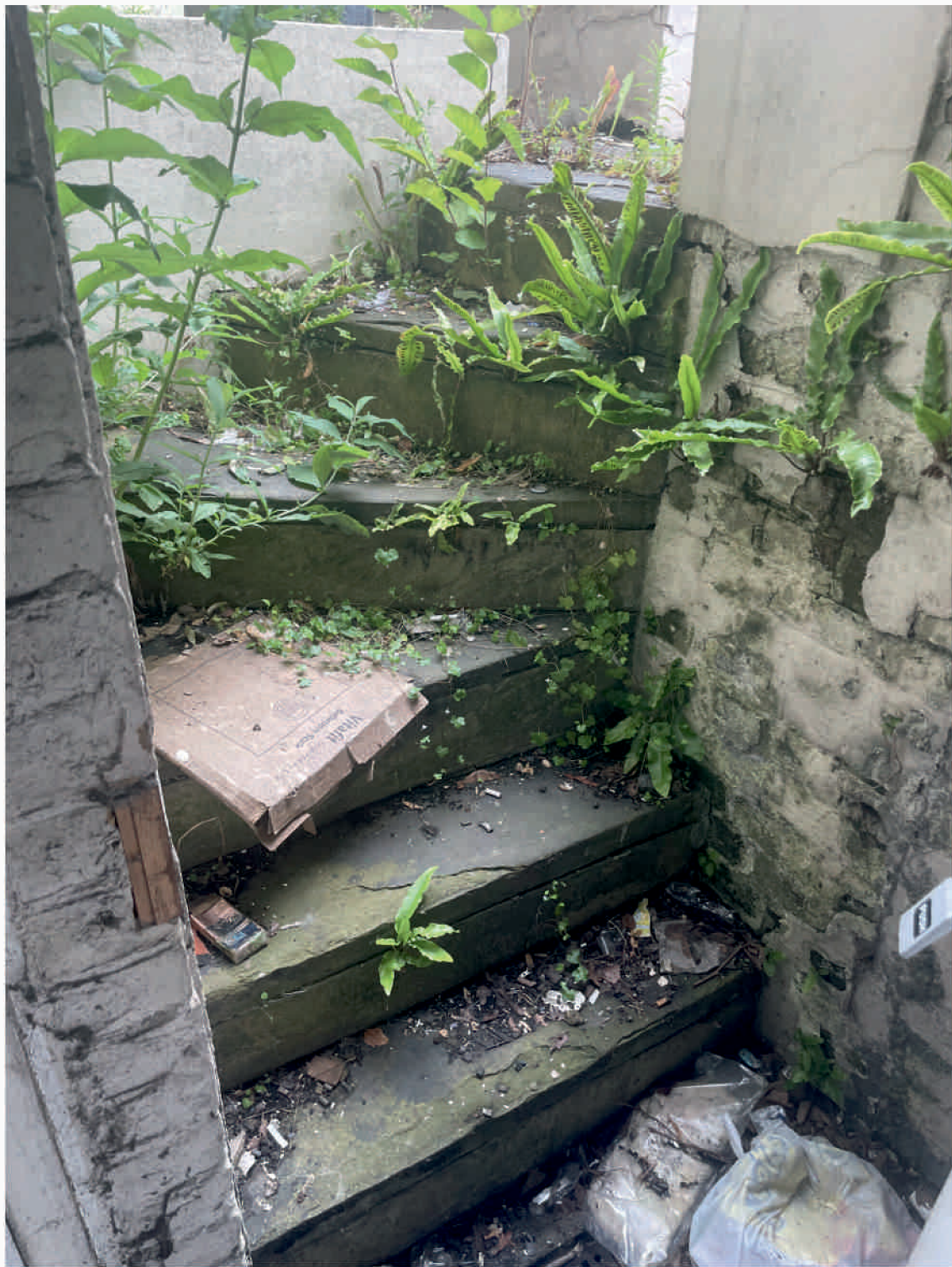
EXTERIOR - Basement steps below entrance stair
