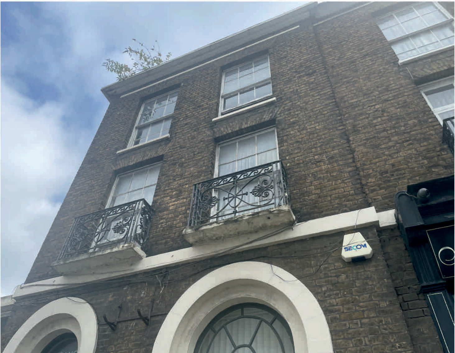
EXTERIOR - Detailed view of upper windows front
