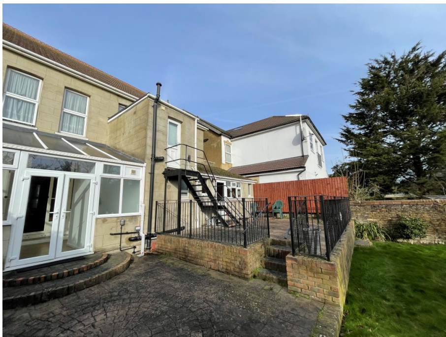
Fig 3 – Rear of No.54 Pelham Road
