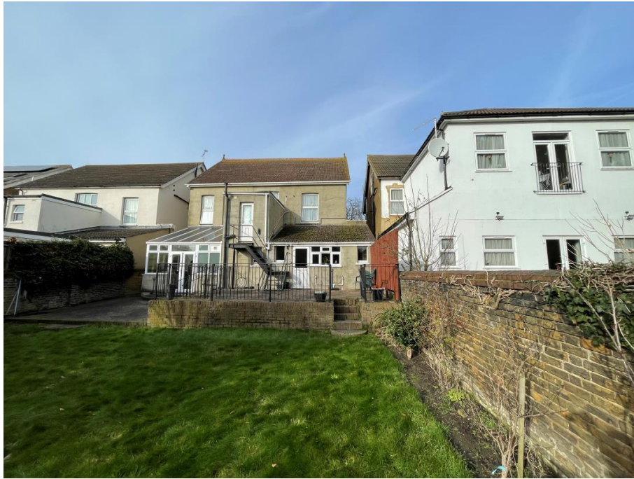
Fig 2 – Rear of No.54 Pelham Road
