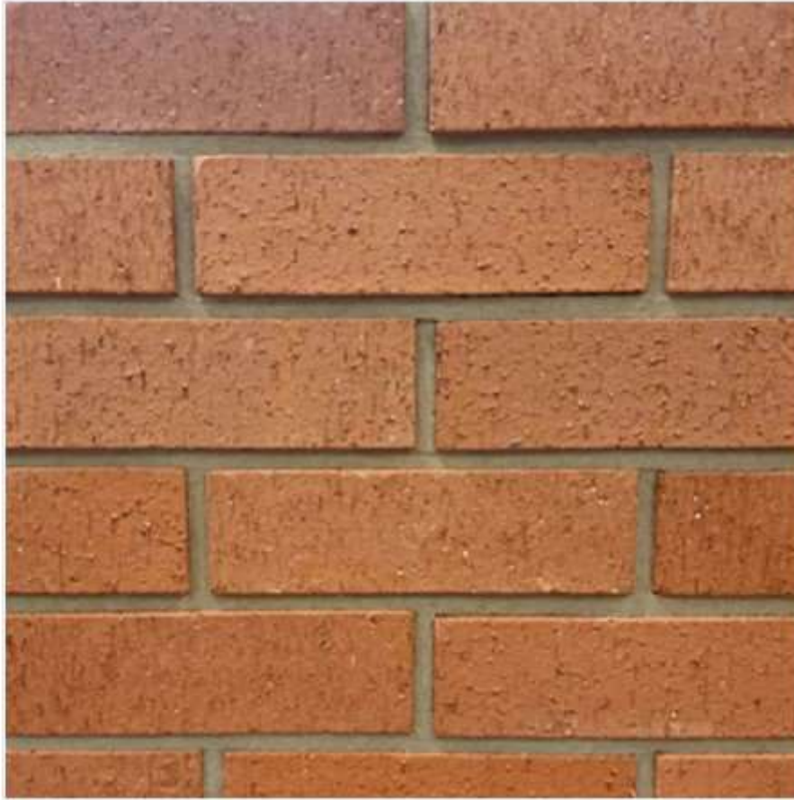
Wienerberger Buxton Red Dragwire 65mm Brick Soldier course above ground floor windows and 150 mm plinth course at base of ground floor
