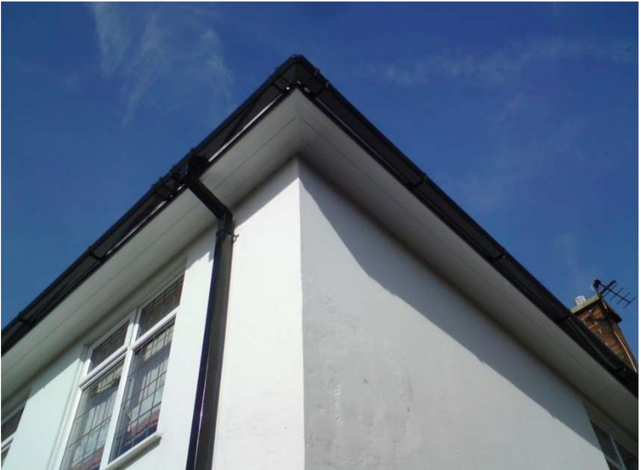
Black upvc guttering and downpipe with white upvc fascia and soffit
