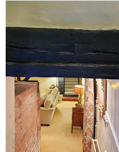
Beam above inserted C19th stair (photographed walking down to living room)
