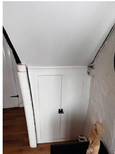
Inserted C19th stair and cupboard to be removed (dining room location)
