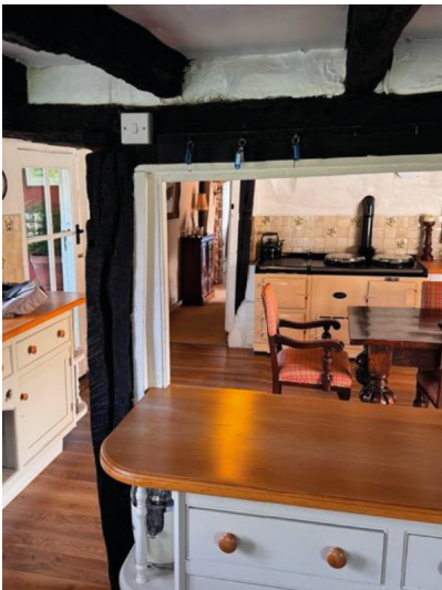
Partition dividing kitchen to be fully reinstated with infill (viewed from kitchen)
