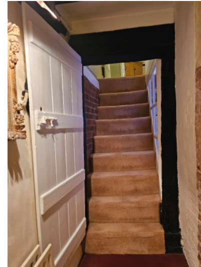
Inserted C19th stair and door to be removed (viewed from living room)
