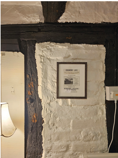
Close up of partition dividing kitchen (viewed from kitchen)
