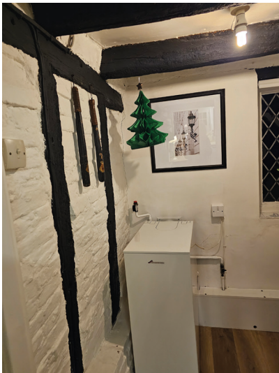
Partition to be altered to create new door opening (from utility room)
