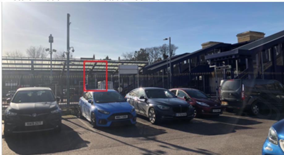
Photo of Platform 2 from Station Car Park
