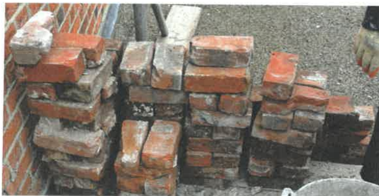
P001 – reclaimed bricks and saved bricks to be used for reconstruction available on site for inspection.
