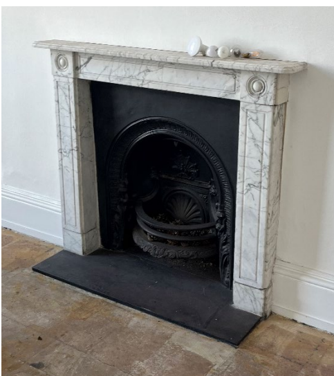
Front view of fireplace.
