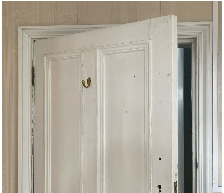
Examples of varying original architraves to be retained across the main house.
