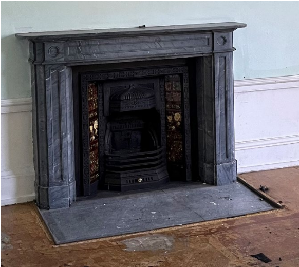
Images of fireplace to Unit 5.
