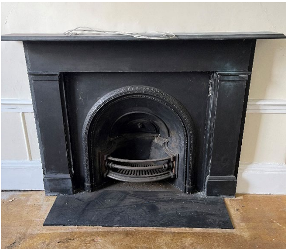
Front elevation to fireplace to Unit 6.
