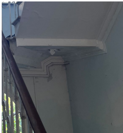
Staircase cornice details found on the main staircases throughout the main house.
