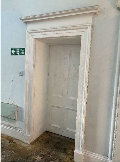
Original doors and architraves on landing of main staircase to remain but become fixed shut with wall behind.
