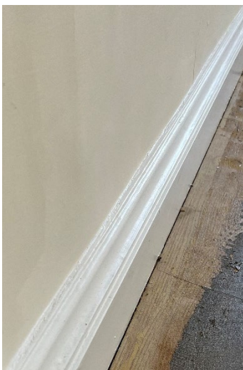
Images of existing original skirting profile, to be retained and repaired.
