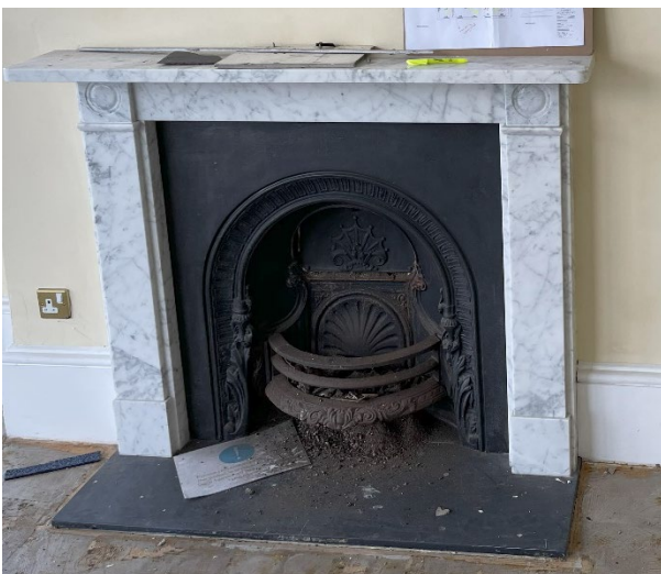
Front view of fireplace.
