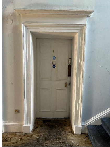
Original doors and architraves on landing of main staircase to remain but become fixed shut with wall behind.
