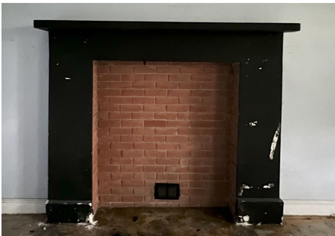
Front elevation of fireplace surround.
