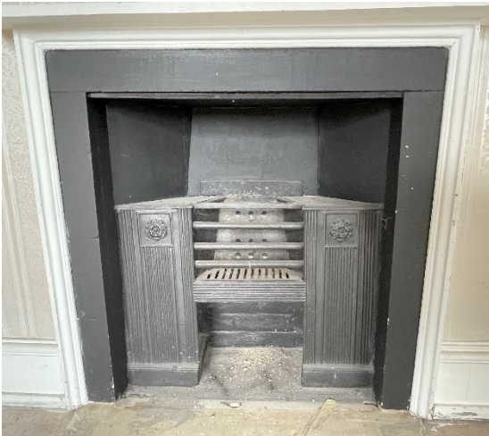
Close up of early 19 th century grate.
