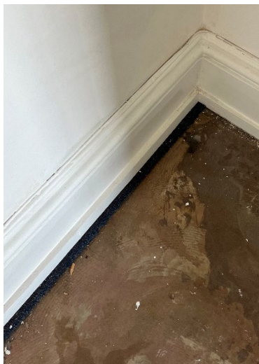
Images of existing original skirting profile, to be retained and repaired.
