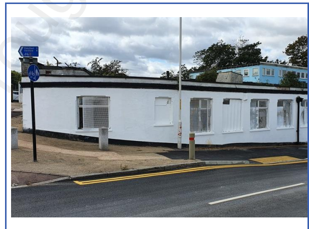
View of the building on site looking south-west across The Shore
