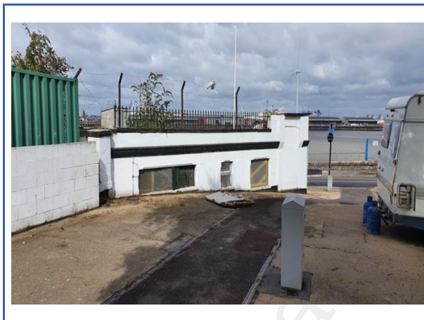
View of the building on site looking north towards the River Thames
