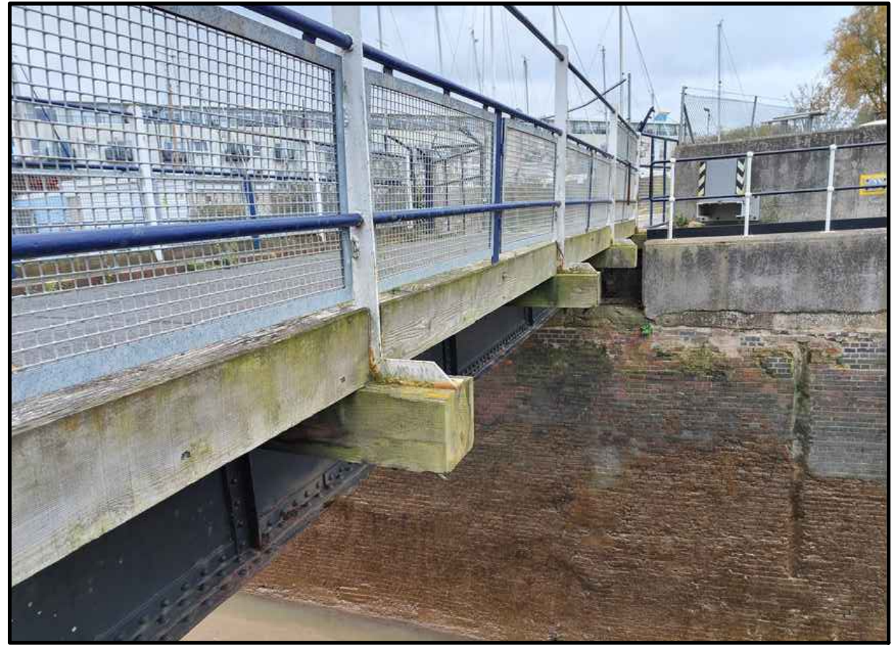
PHOTO 1 - ELEVATION TO SIDE OF EXISTING BRIDGE
