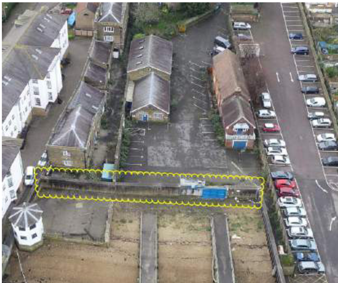
Photograph 2.0 - Existing steel sheet piled wall, encased in concrete and clad in masonry
