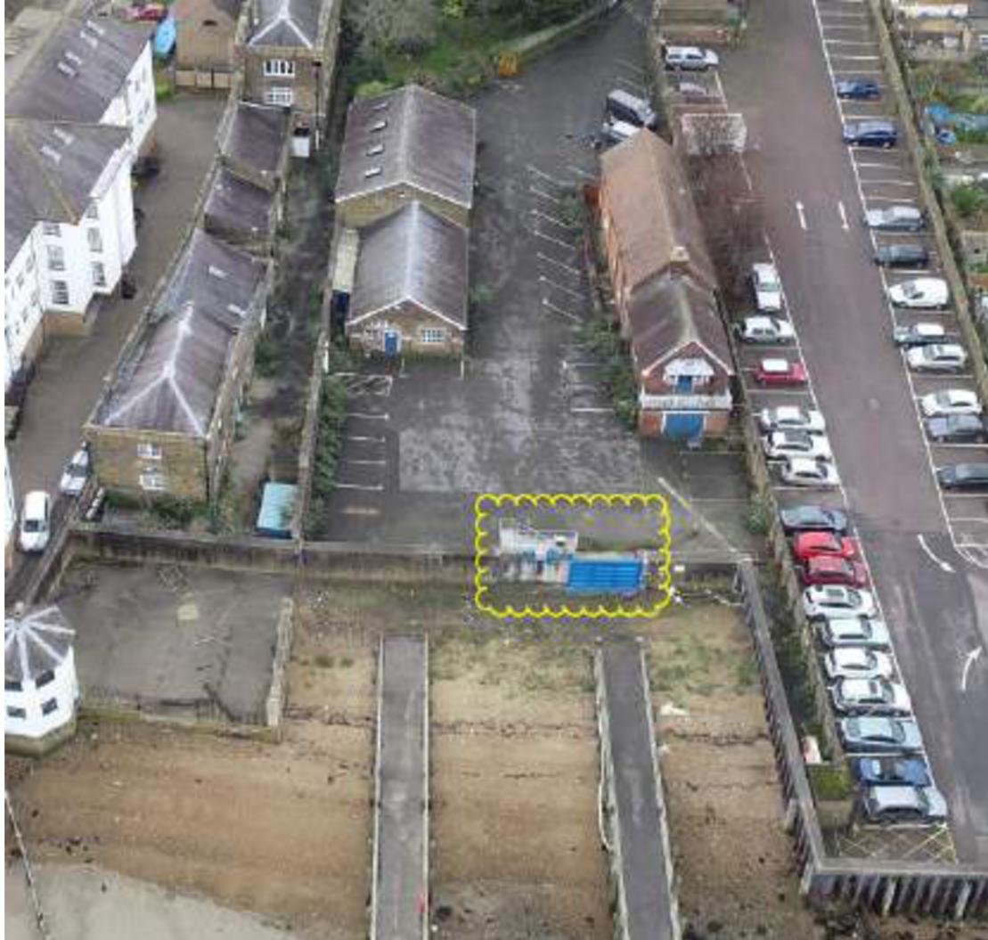
Photograph 3.0 Flood gate and stair location
