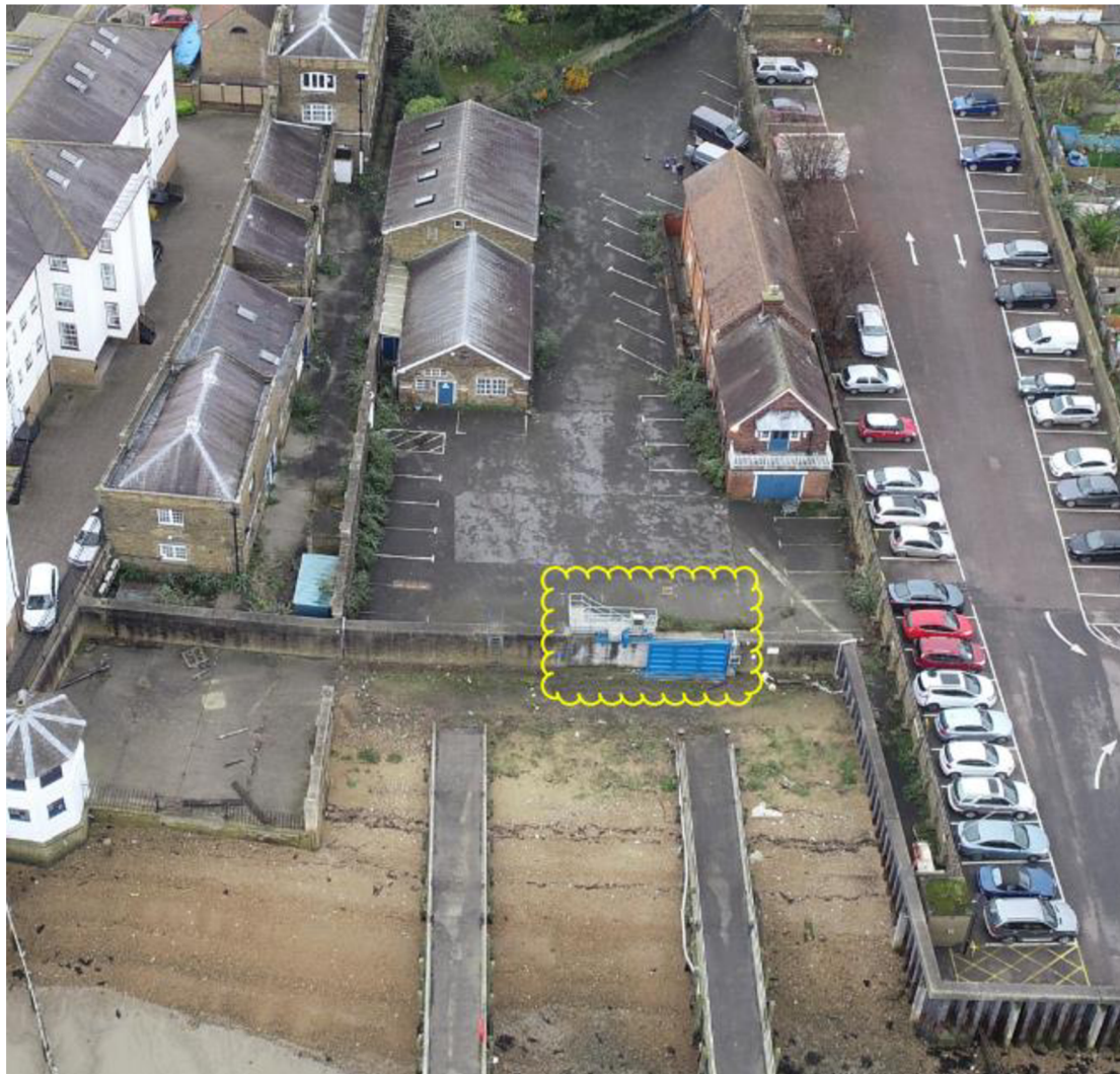
Photograph 3.0 Flood gate and stair location
