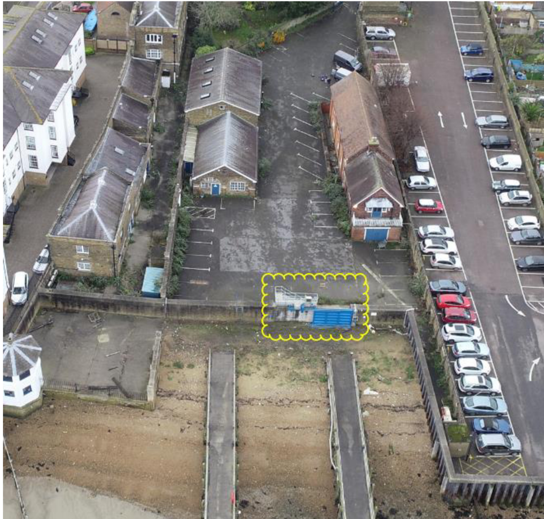
Photograph 3.0 Flood gate and stair location
