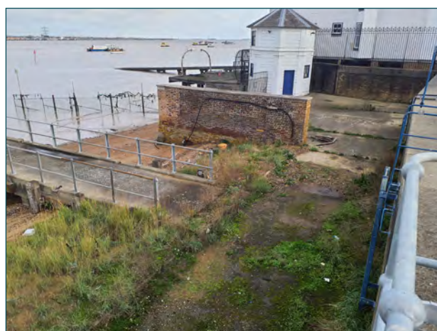
Photograph 4. Areas of hardstanding and coastal vegetation along the northern boundary.
