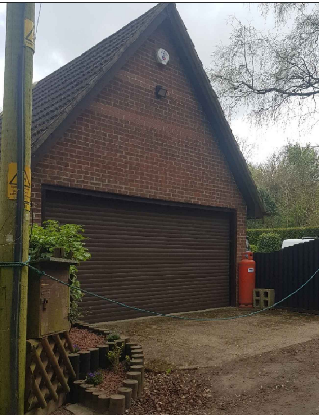
Pitched garage. Approx 5.7m high
