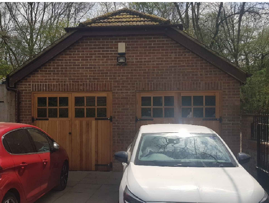
Copperfield existing garage 4.8m high
