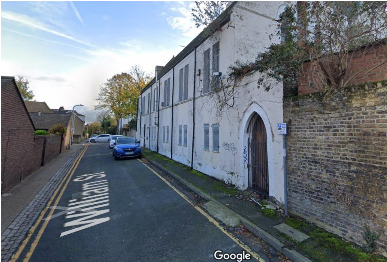
Fig.4 Rear view of property looking east along William Street.
