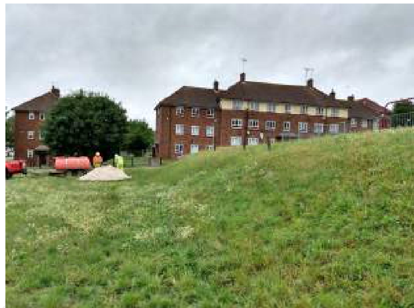
Slope to western end of site
