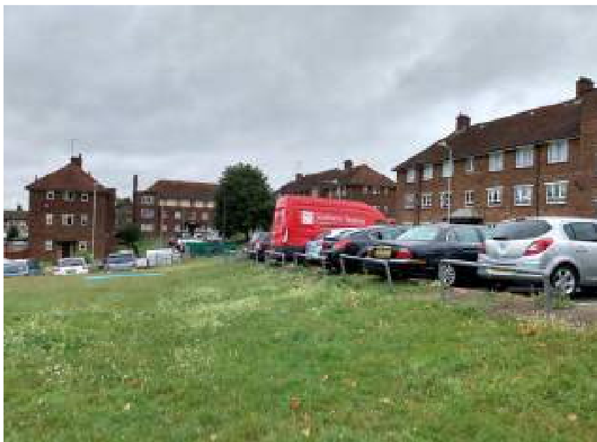
Eastern end of site to north east
