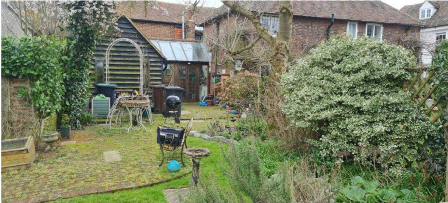
Photo 4: Photograph 2: West facing elevation of 30 The Street
