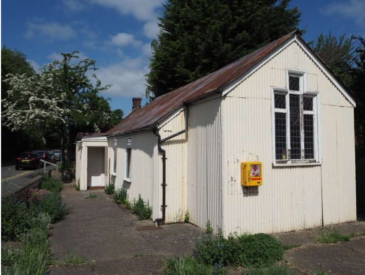
Sole Street elevation (from the south-east)
