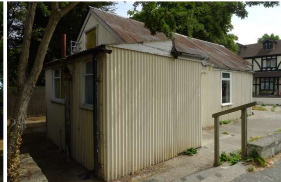
South-west corner with existing extension block
