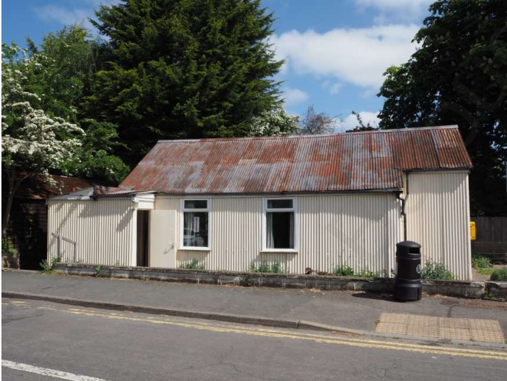
Manor Road elevation (from the south)
