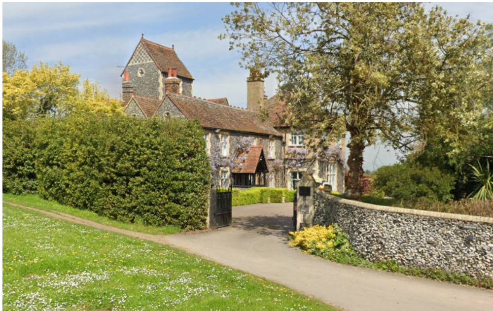
P002 – entrance area looking into site
