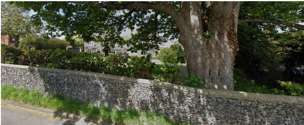
P010 – forge lane view to east elevation from road
