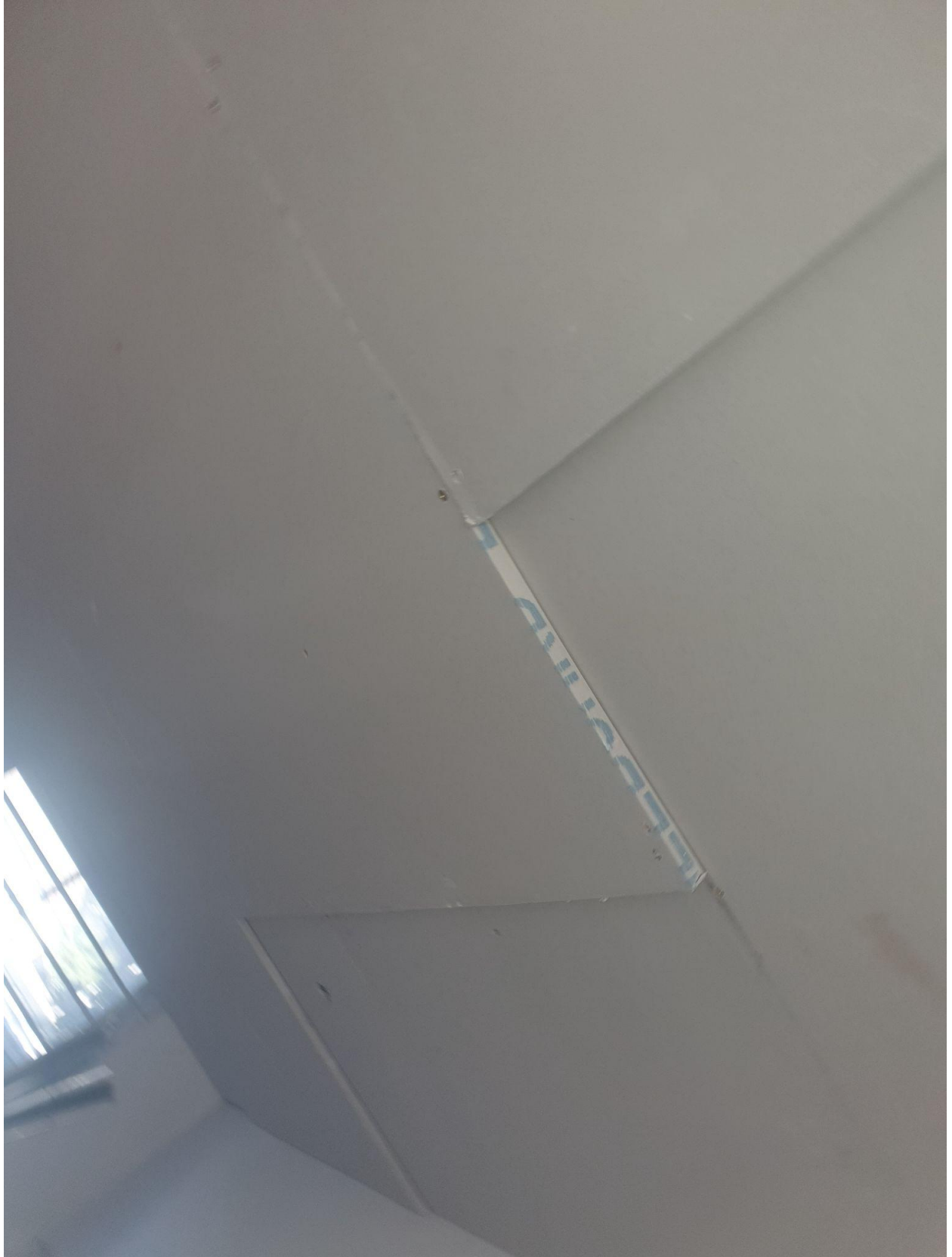
Double layer plasterboard tacked to mfc ceiling with staggered joints
