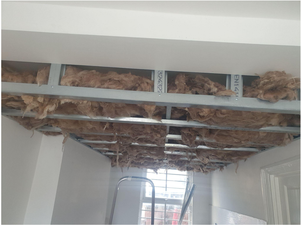
100mm rockwool insulation fitted above mfc ceiling
