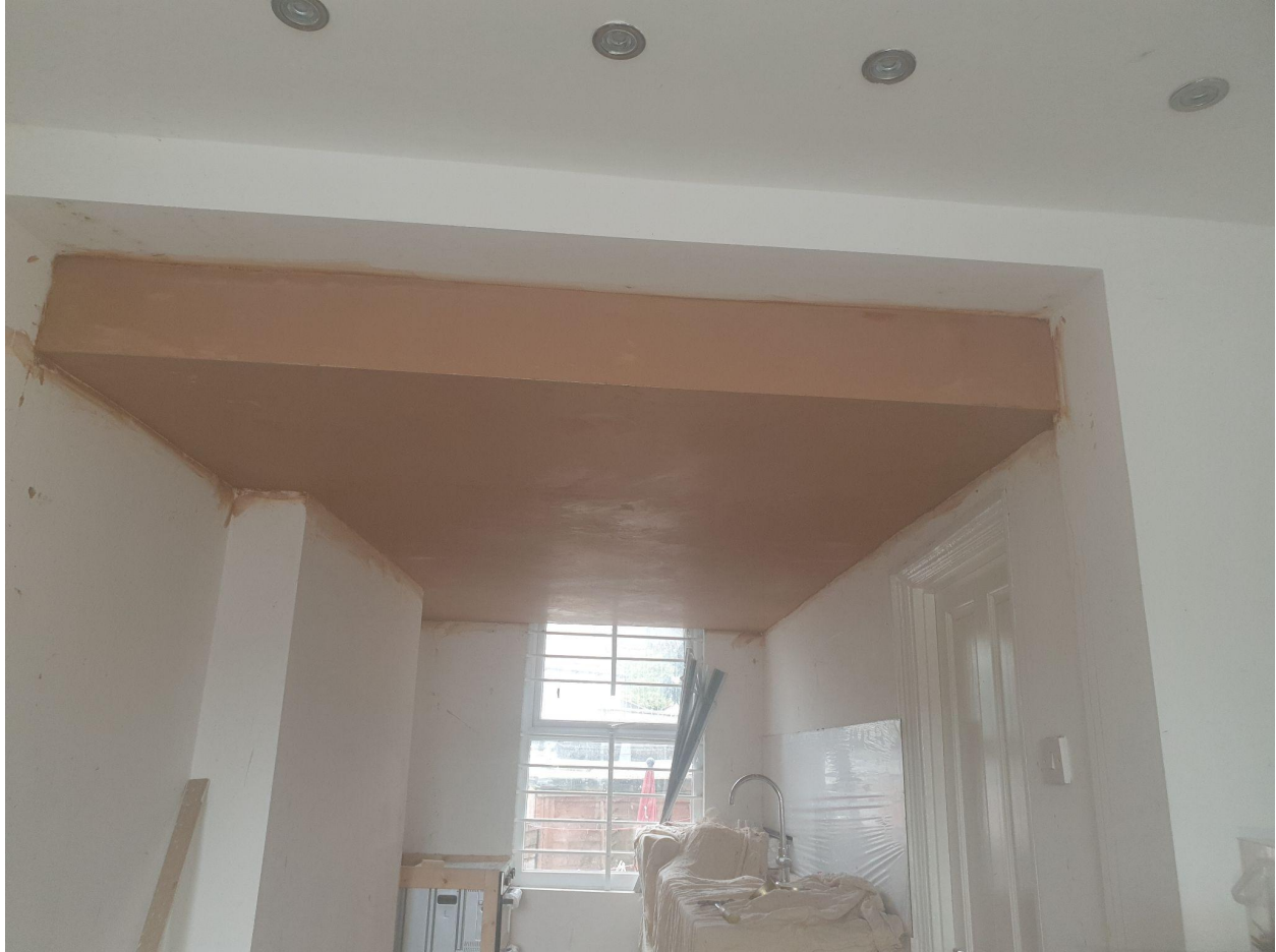
New plasterboard ceiling taped and skimmed with gyproc multifinish
