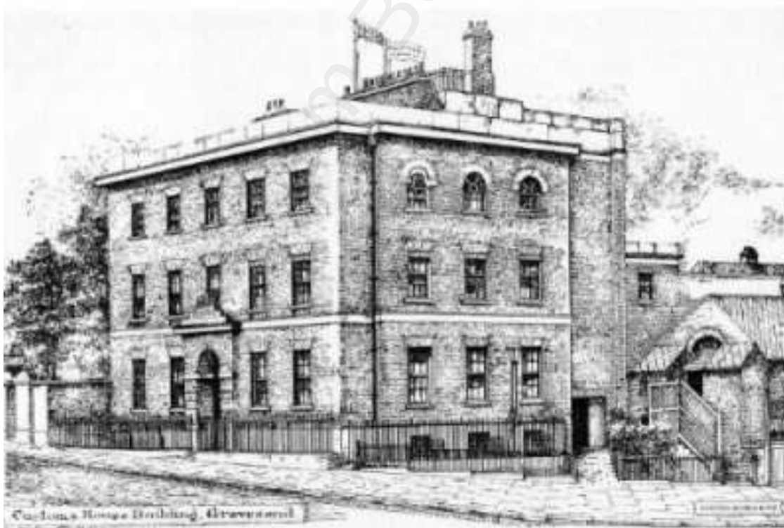
Fig 12 A matching drawing of the Customs House of the same date owned by D Grierson: a pen and ink drawing by Llwyd Roberts in Historical Walk Through Gravesend and Northfleet 1935 , partially showing the roof lookout and the buildings on the eastern boundary. The view is remarkably unchanged now.
