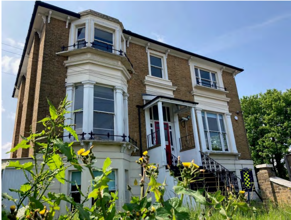
Plate 1: St Joseph's Convent Preparatory School, view of three storey late - 19 th century building fronting onto Old Road East (looking south)
