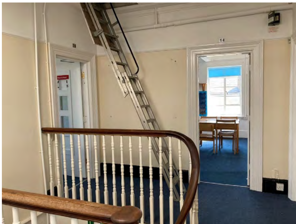
Plate 6: St Joseph's Convent Preparatory School, view the 2nd floor landing within the late-19 th century building (looking north/north-west)
