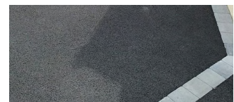
Entrance Road Asphalt
