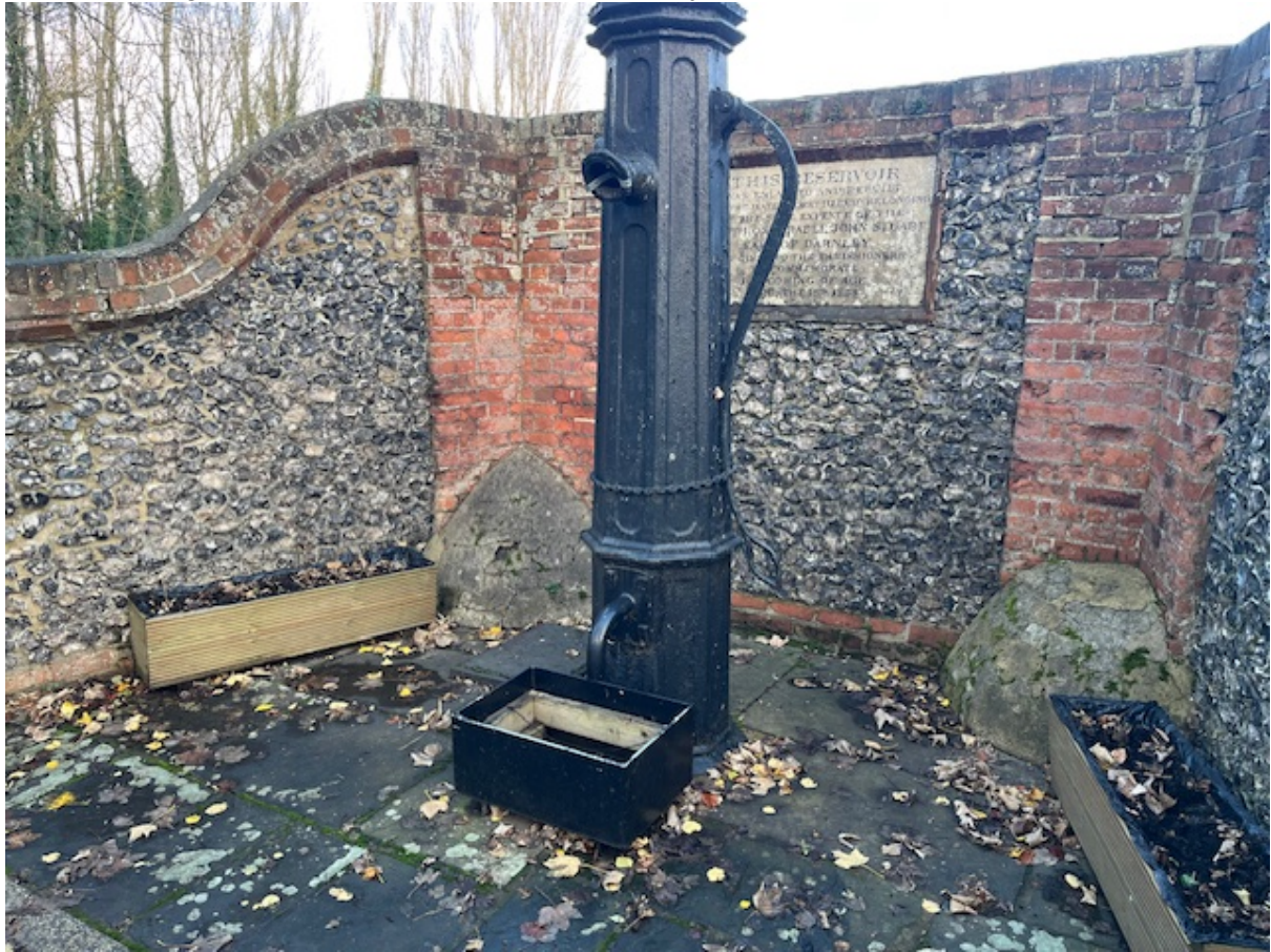
Cobham village pump wall Maintenance works only
