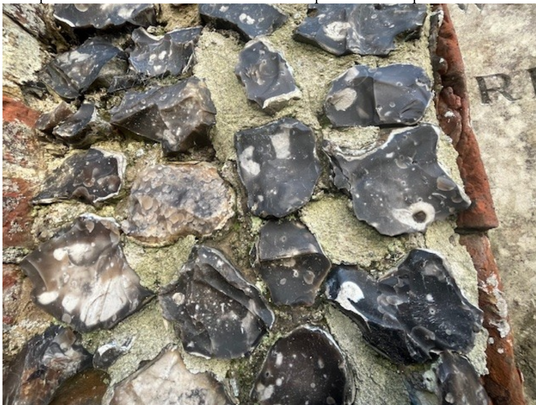
Examples of cement mortar to be removed and repointed in flint panels and brickwork
