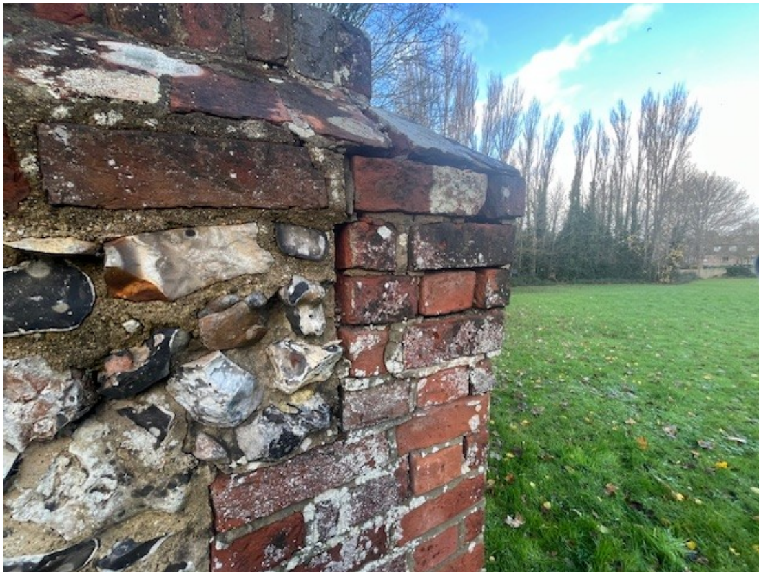
Examples of cement mortar to be removed and repointed in flint panels and brickwork
