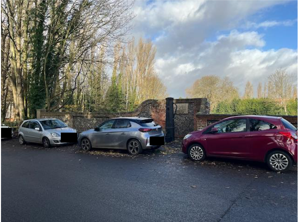
Wall View from front
