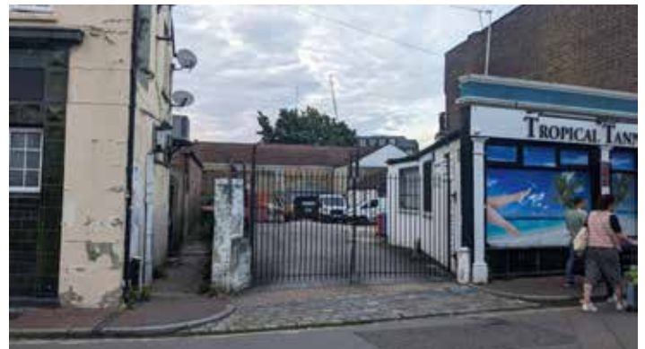
Views through to industrial yards and unlawful shopfronts. South side of the road.
