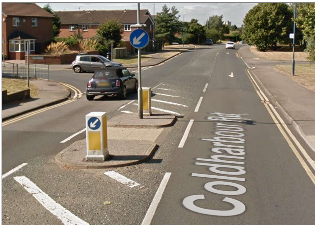
Figure 3-4: Uncontrolled Crossing Located along Coldharbour Road
