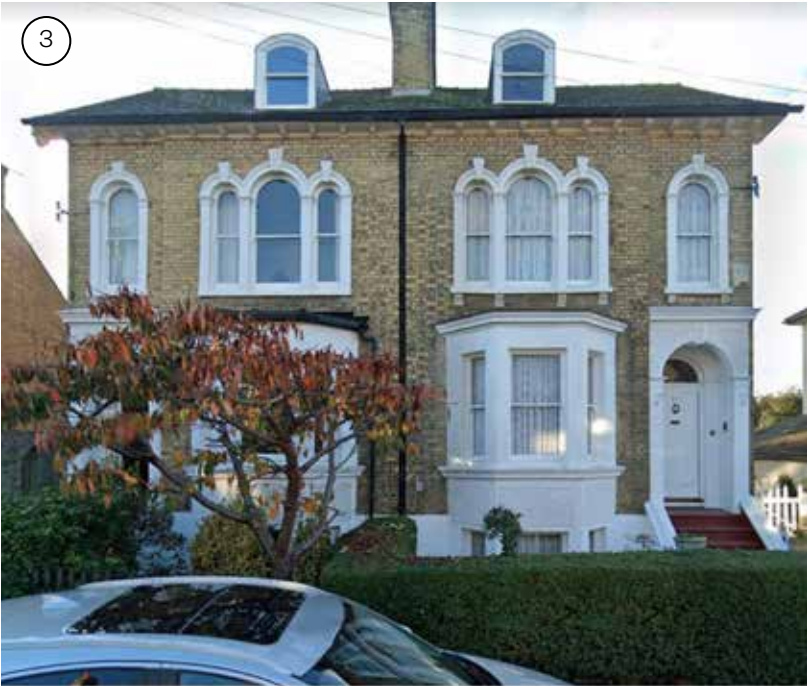
Whitehill Road - Victorian style
