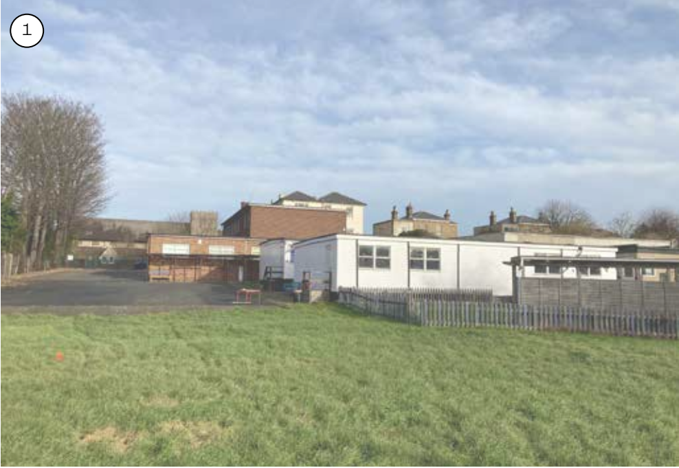
View facing entrance into the site
