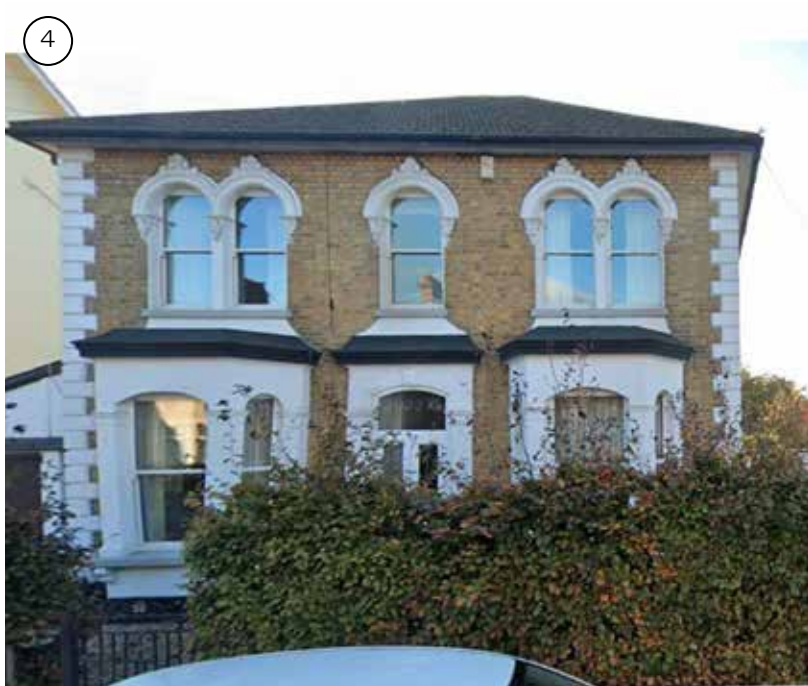
Whitehill Road - Victorian style
