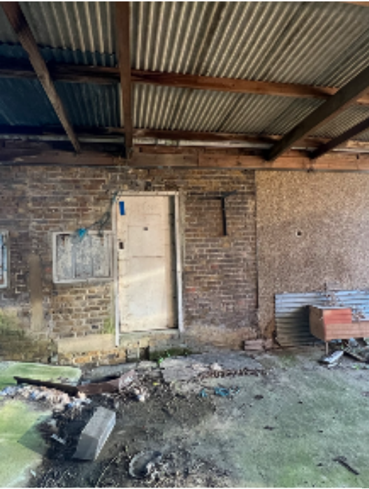
looking at the east elevation from inside, towards building A
