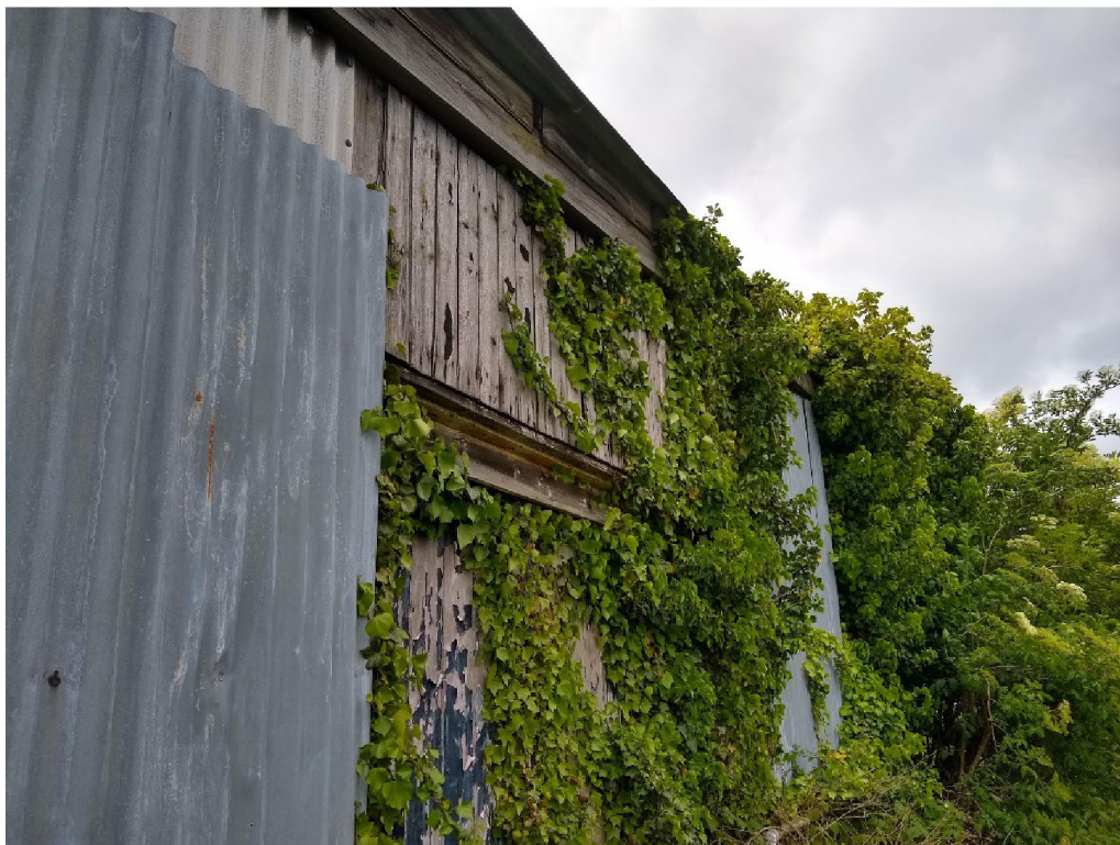
Photo 12 – Building C – north elevation.
