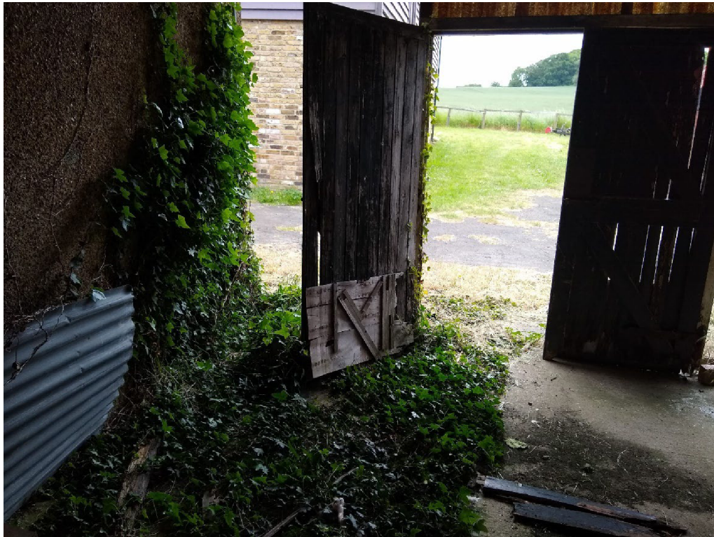
Photo 9 – Building C – internal view of south wall.
