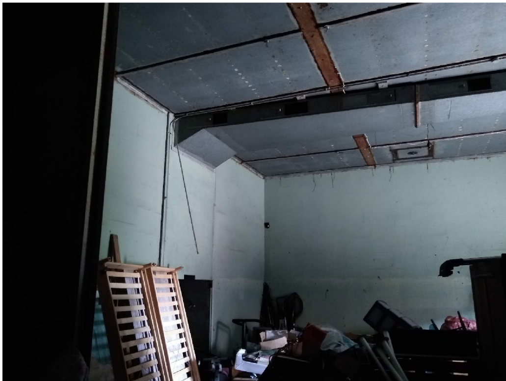
Photo 8 – Building B - internal.
