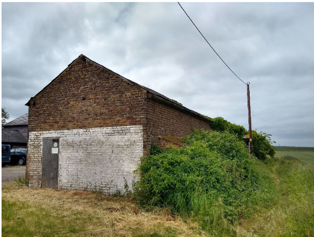
Photo 4 – Building A – east elevation.
