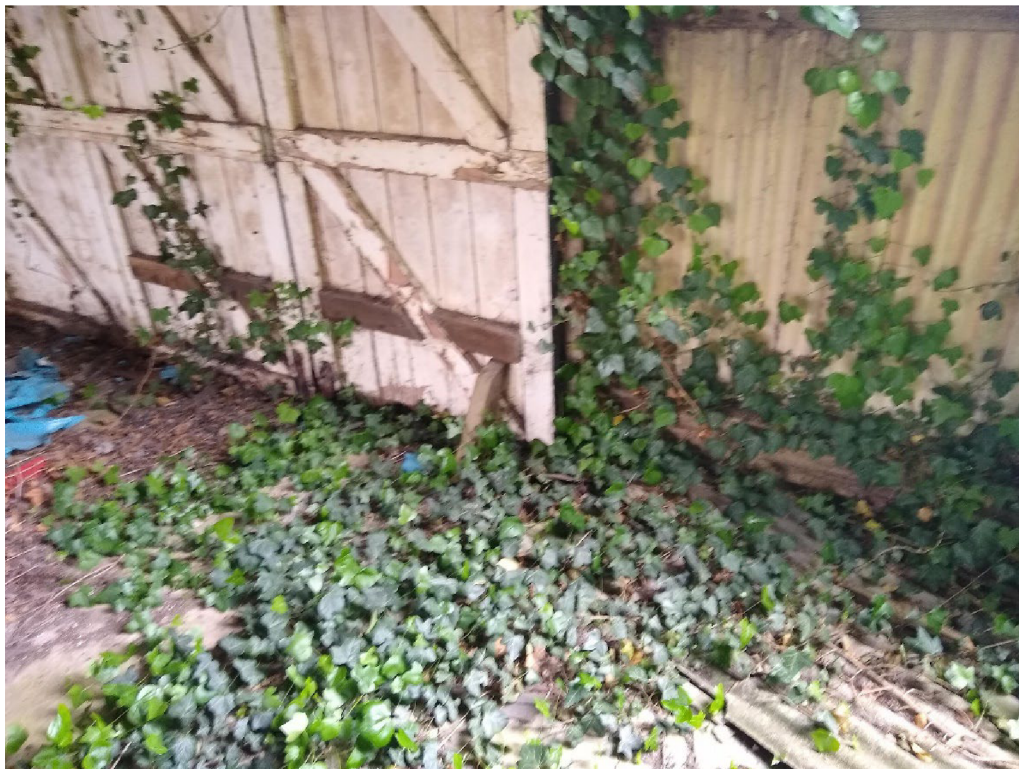
Photo 10 – Building C – sliding door to north wall.
