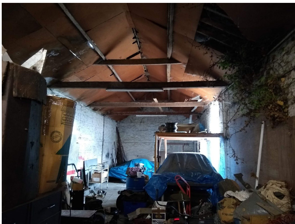
Photo 1 – Building A – internal.
