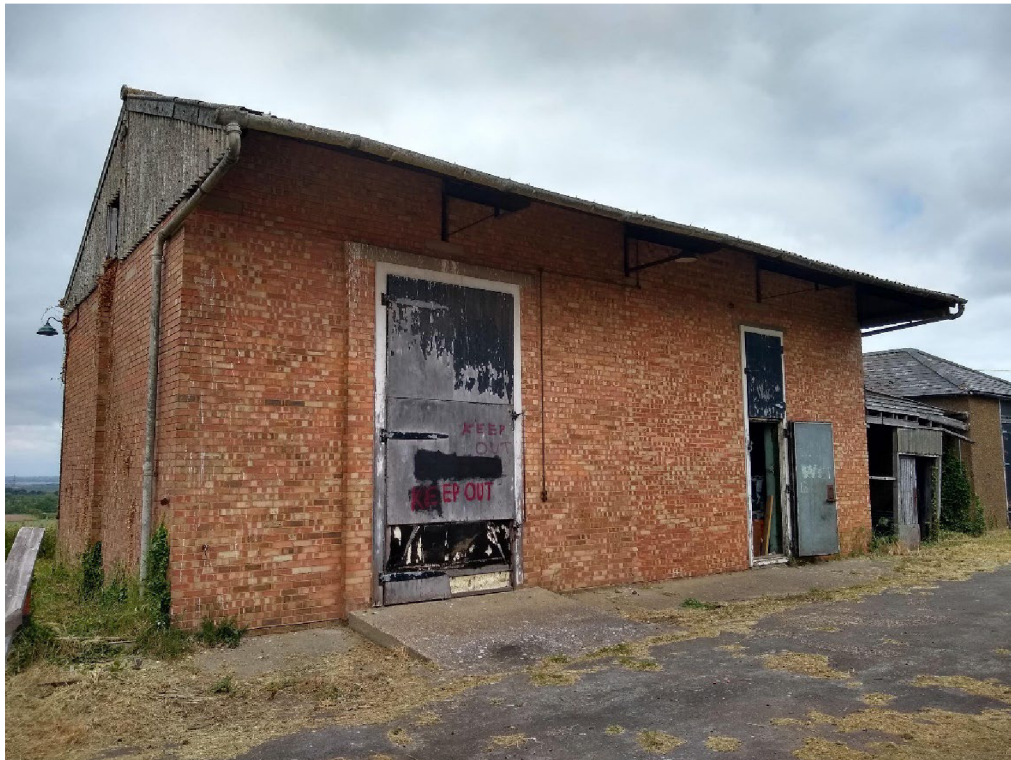
Photo 6 – Building B – south elevation.
