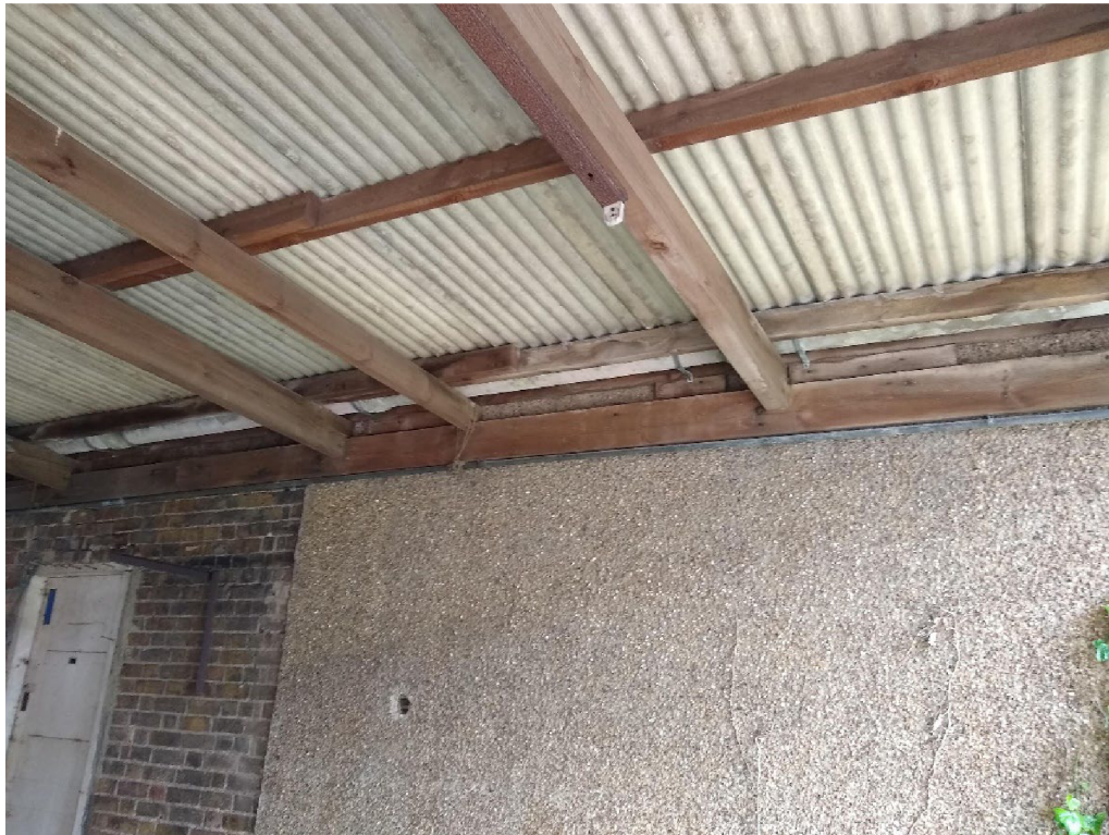
Photo 11 – Building C – roof.
