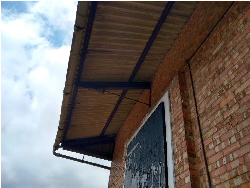
Photo 7 – Building B – canopy overhang.
