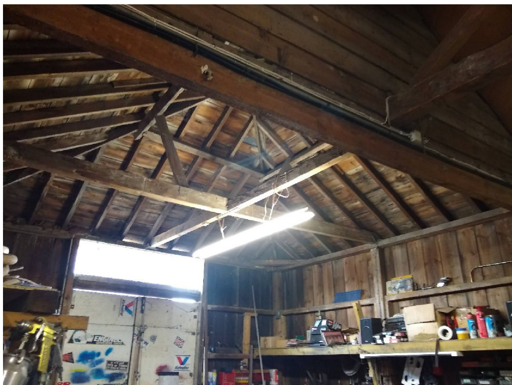
Photo 2 – Building A – internal.
