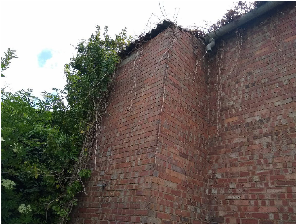
Photo 5 – Building B – north elevation.
