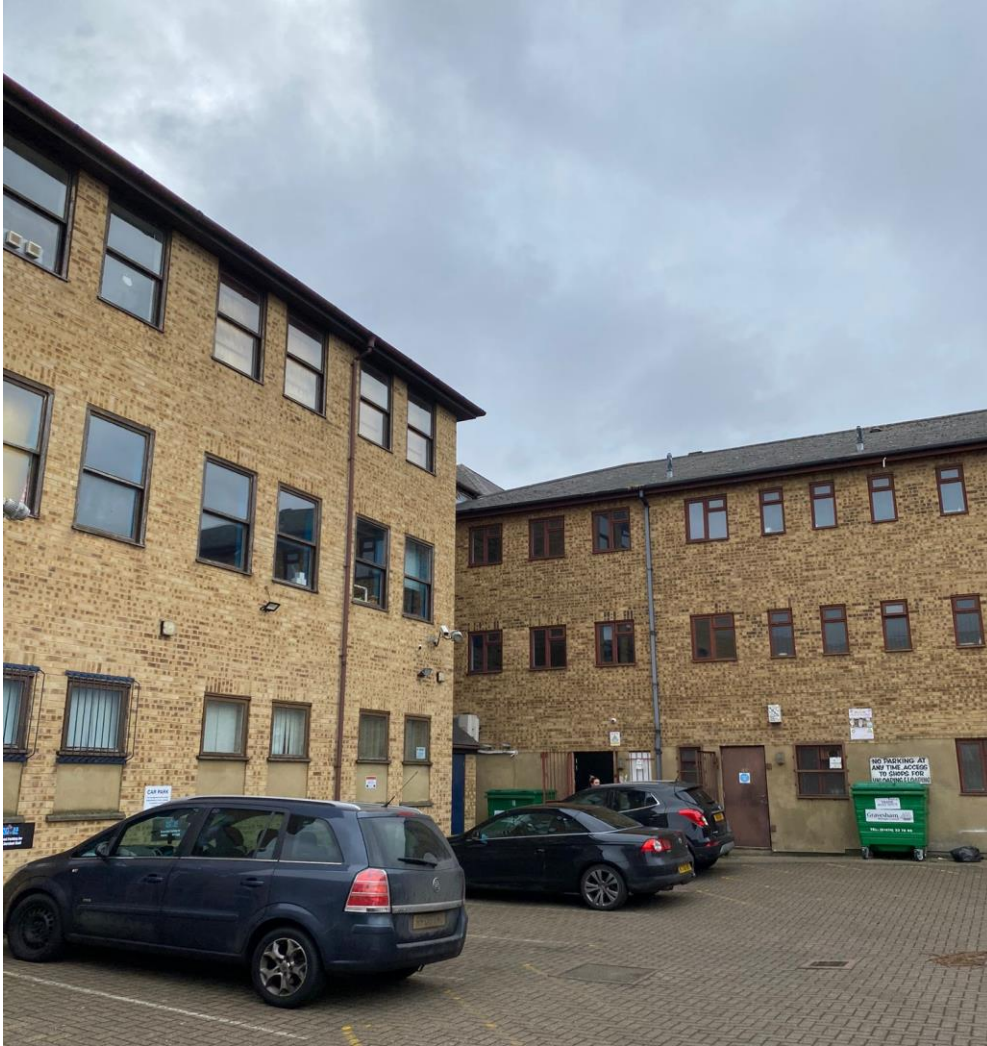
Fig.2: Rear of the property
