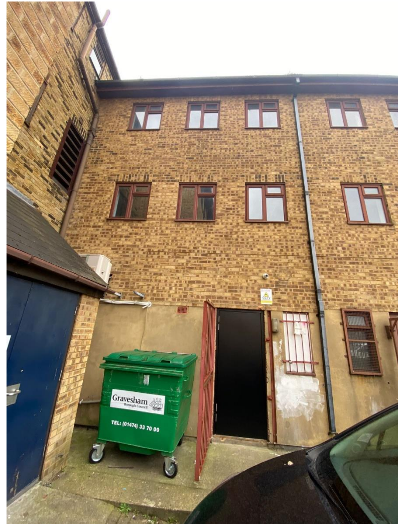
Fig.3: Rear of the property
