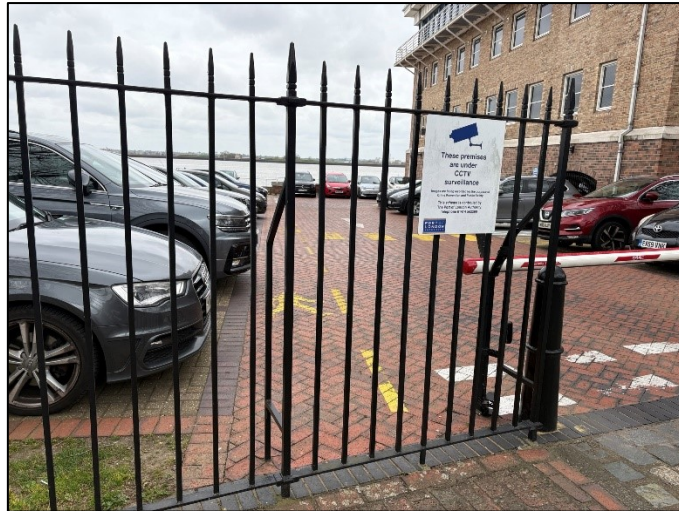
Figure 3: Existing fencing at location of proposed pedestrian gate.
