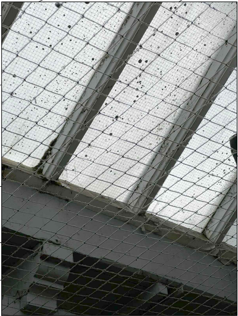
Photo of existing Georgian wire glazing panels to canopy prior to removal.
