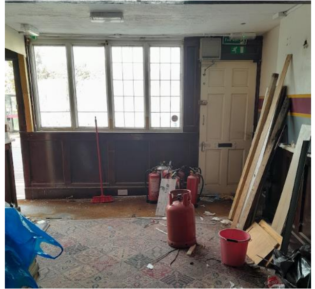
Figure 11. View looking north towards the timber shopfront and main entrance.
