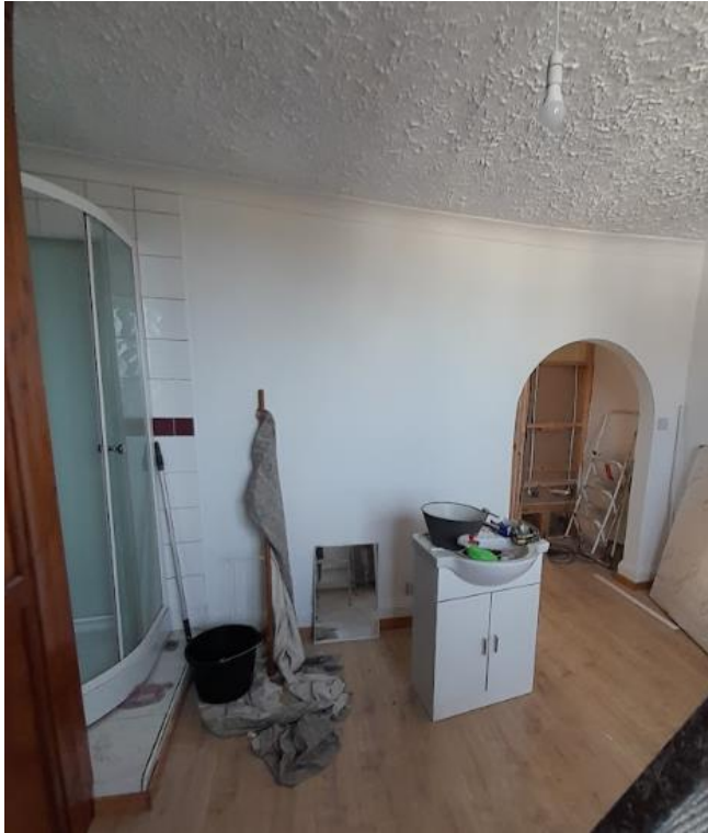
Figure 14. second floor front room illustrating modern ceilings, walls, floor covering and fixtures.
