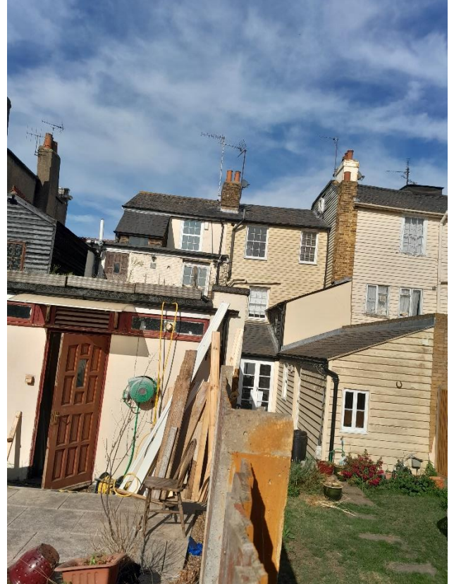
Figure 4: Rear elevations of nos. 44 and 45 (view looking north).
