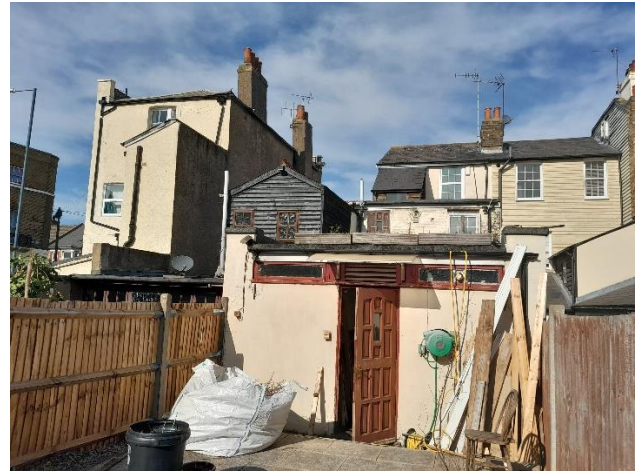
Figure 6: Rear (south) elevations of nos. 42-44 The Terrace.
