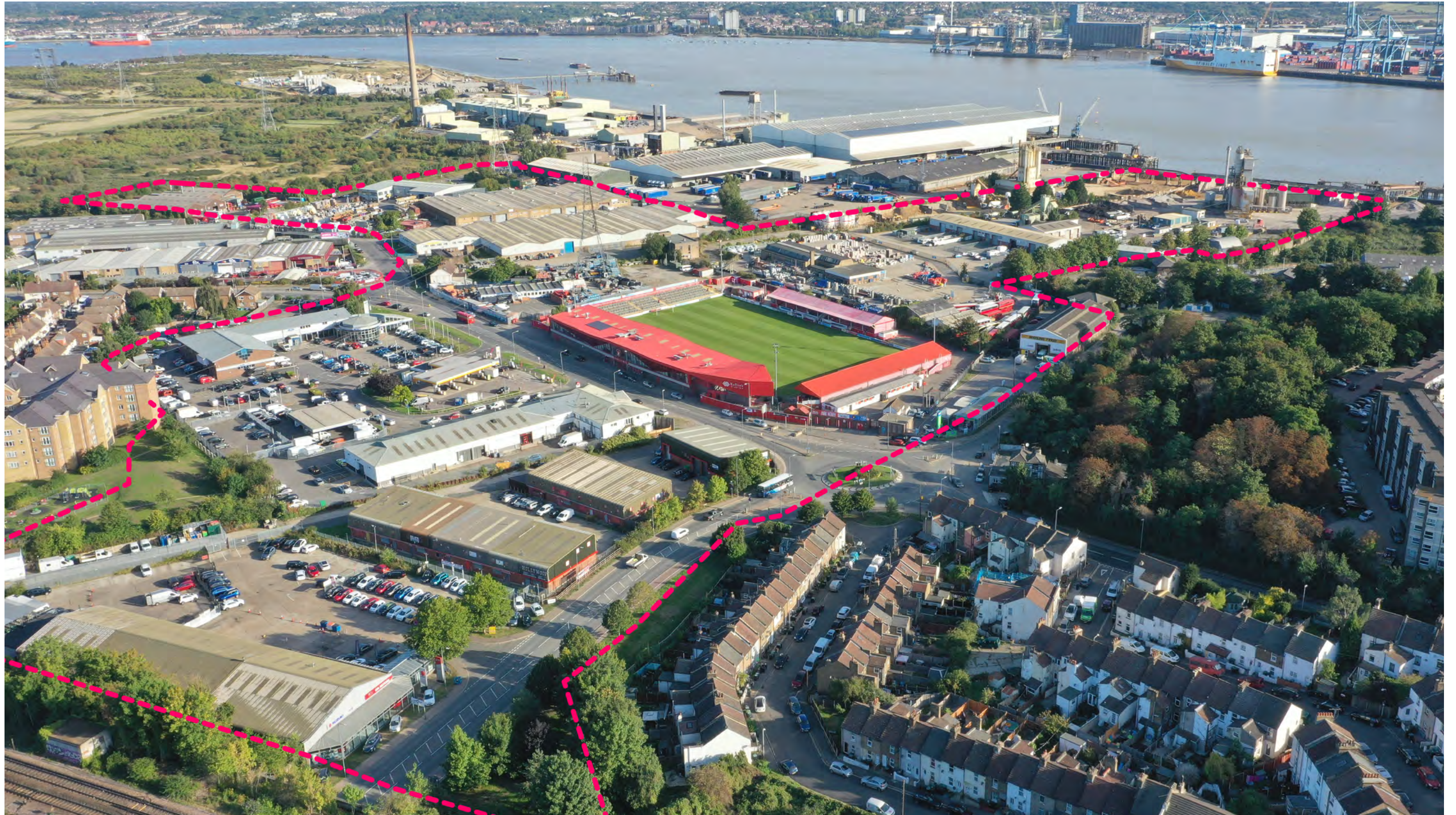
Red line boundary location is approximate in this aerial photograph.
