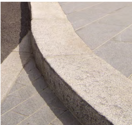
Buff granite kerb stone
