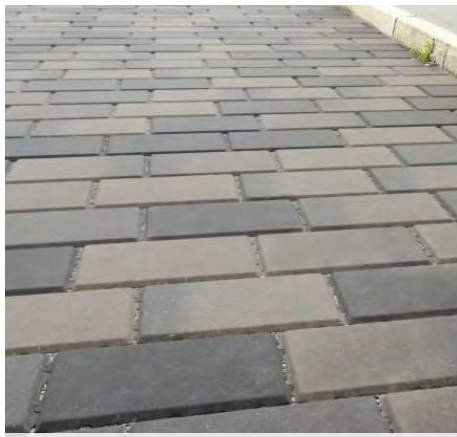
Permeable vehicular sett paving, stretcher bond
