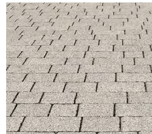
Buff stone pavers, stretcher bond
