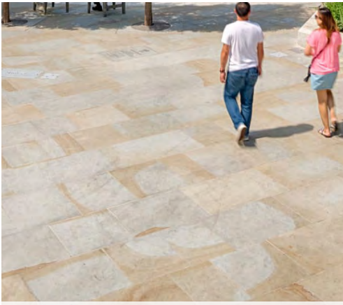
Yorkstone paving flags, stretcher bond
