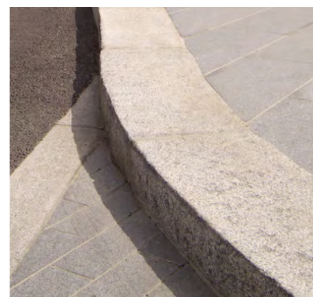
Buff granite kerb stone
