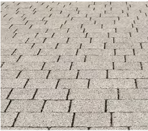
Buff stone pavers, stretcher bond
