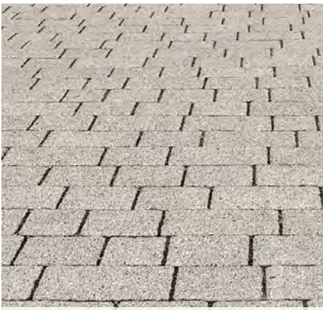
Buff stone pavers, stretcher bond
