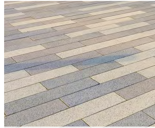
Buff tone rectangular concrete flags, stretcher bond
