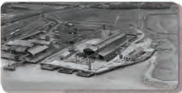
Brittania lead and cement works_ 1933
