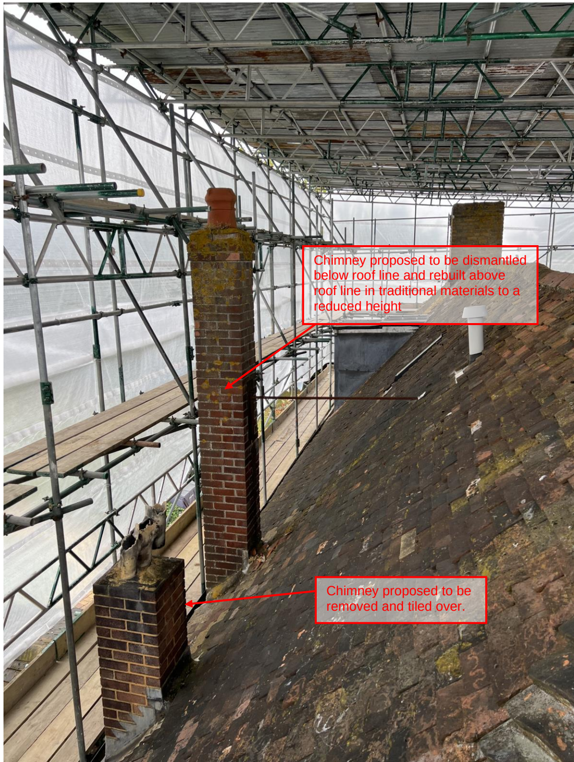
The two rear chimneys of modern construction.
