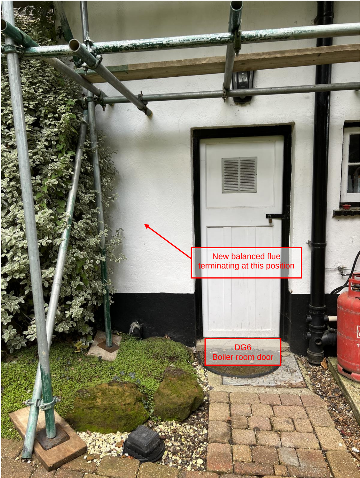
Position of new balanced flue
