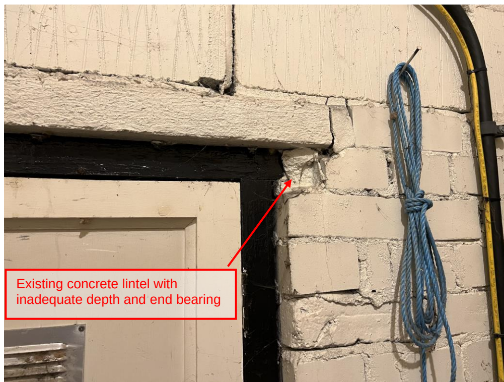
Close-up photo of bearing end of concrete lintel to be replaced
