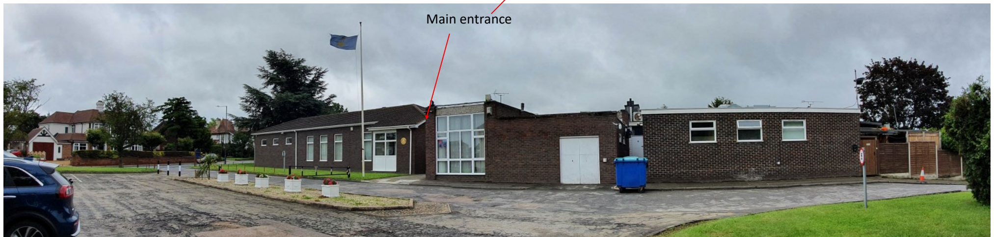
Fig 9—Front view of Clubhouse
