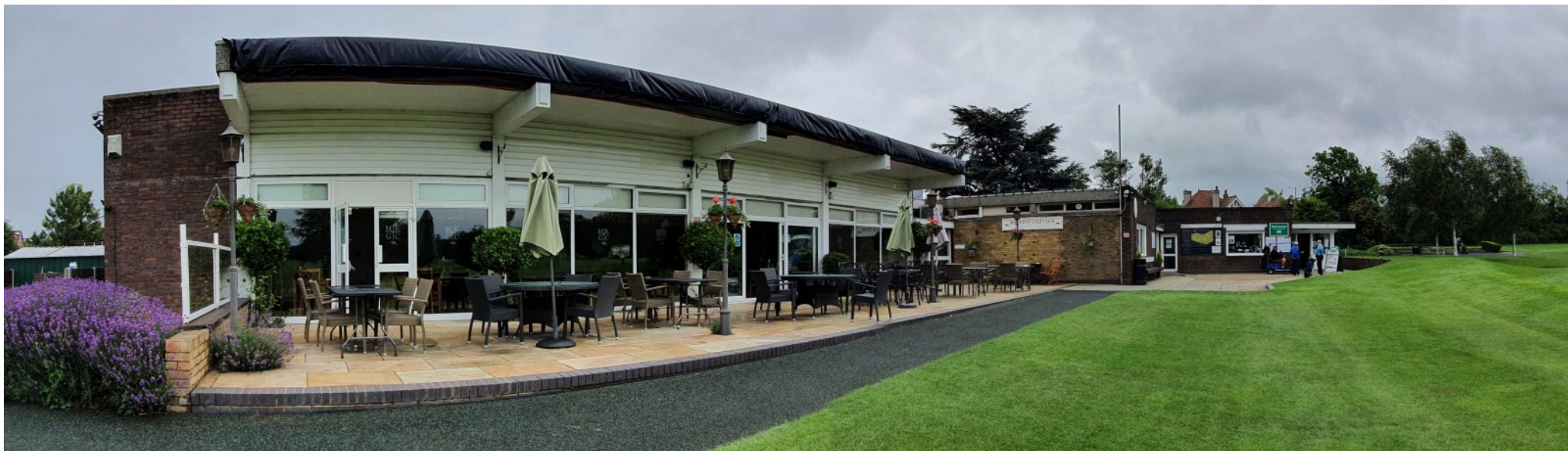
Fig 11—Rear view with the Bar/ Lounge terrace in the foreground
