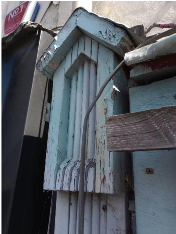
Left-hand shopfront pilaster with reeding detail
