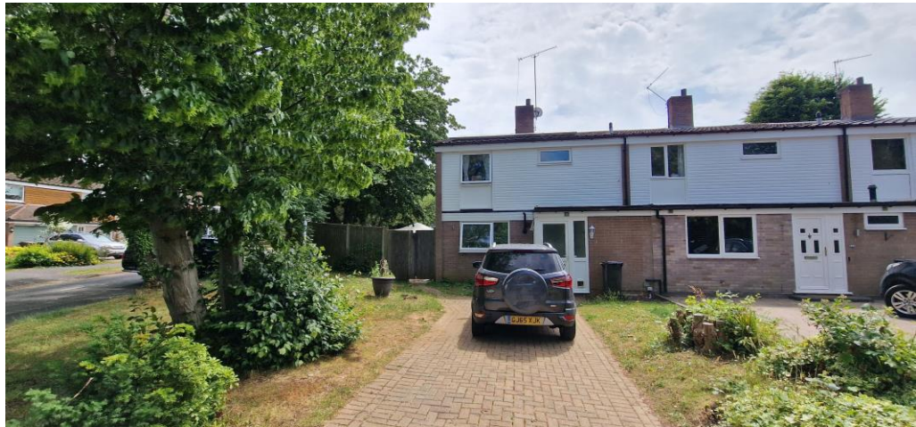
51 Timber Bank as viewed from North
